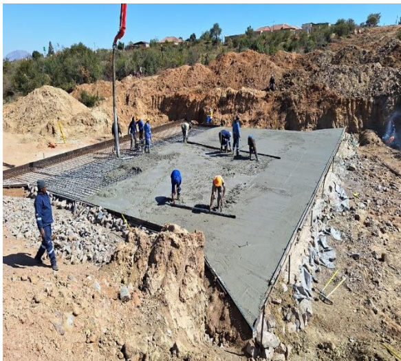
Bridge linking Matobole and Molatela
