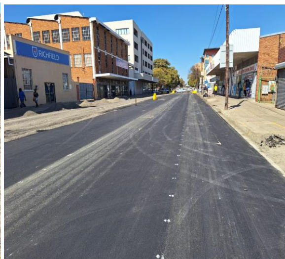
Rehabilitation of church street
