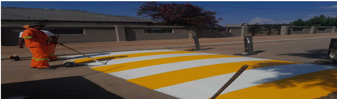
Routine maintenance (Speed hump marking)
