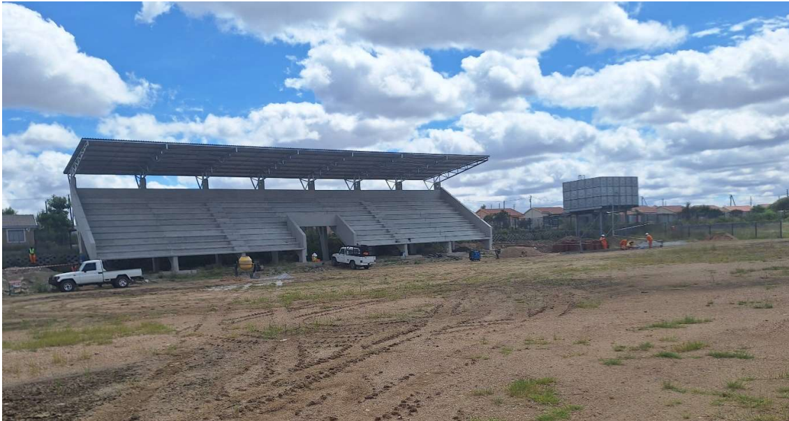
Ext 44/78 Construction of Grandstand 2024
