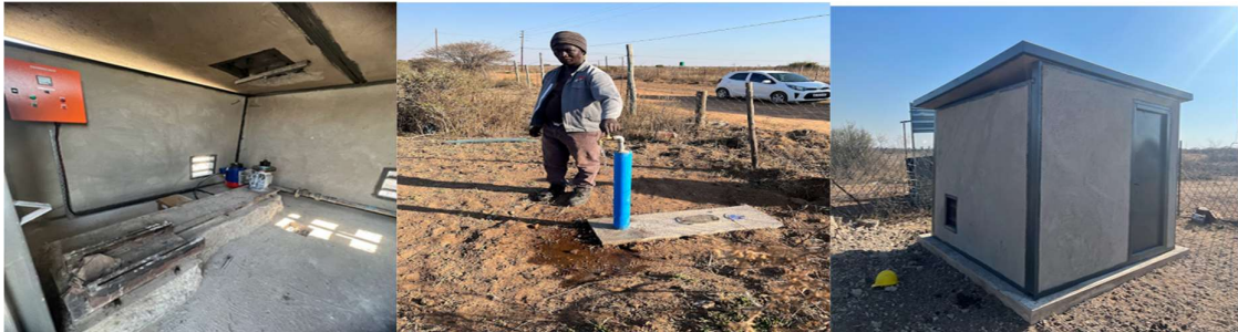
Mars Phase 1 with 82 Yard connections installed
