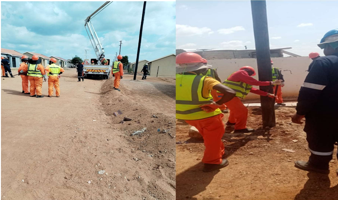
Pictures during construction
