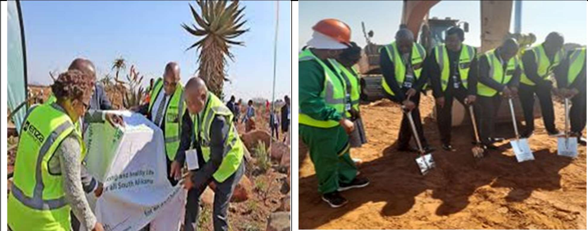
Health Minister, Dr Joe Phaahla, and other government officials turned the first sod to mark the birth of the ground-breaking new Limpopo Central Hospital
