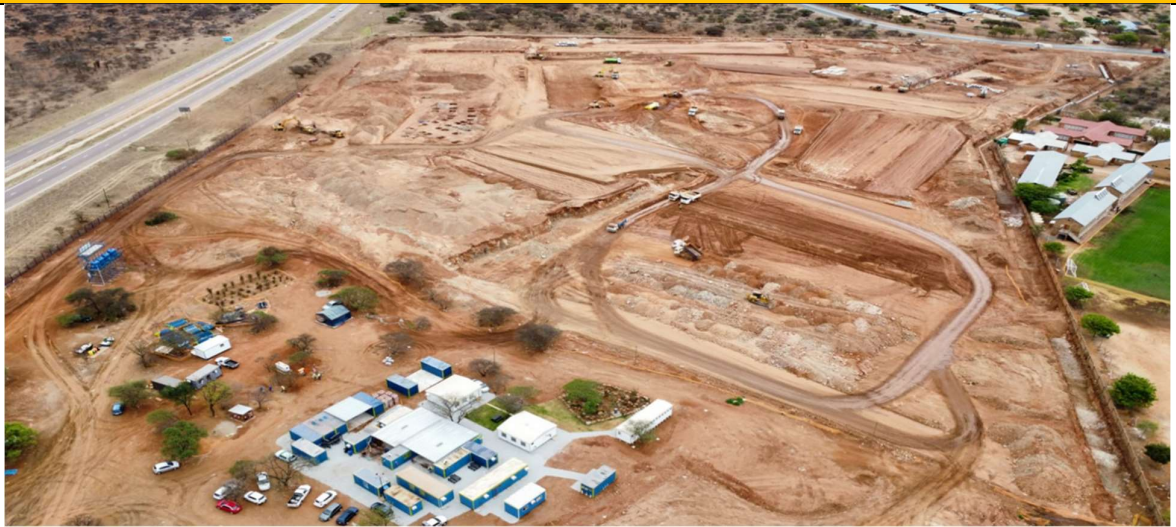
Bulk Underground Services Installation
