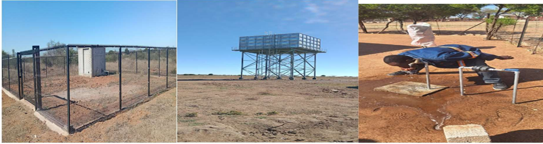
Magodu Phase 1 with 36 Yard connections installed
