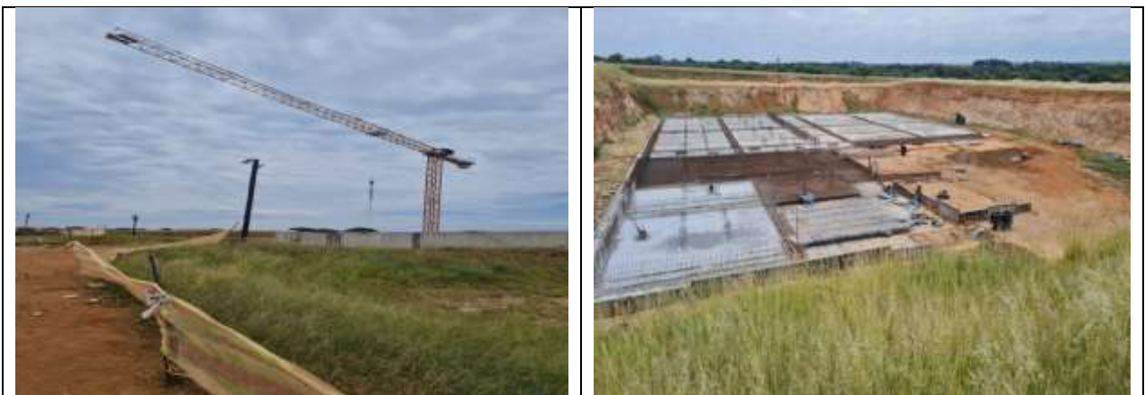
New Regional Wastewater Treatment Plant
