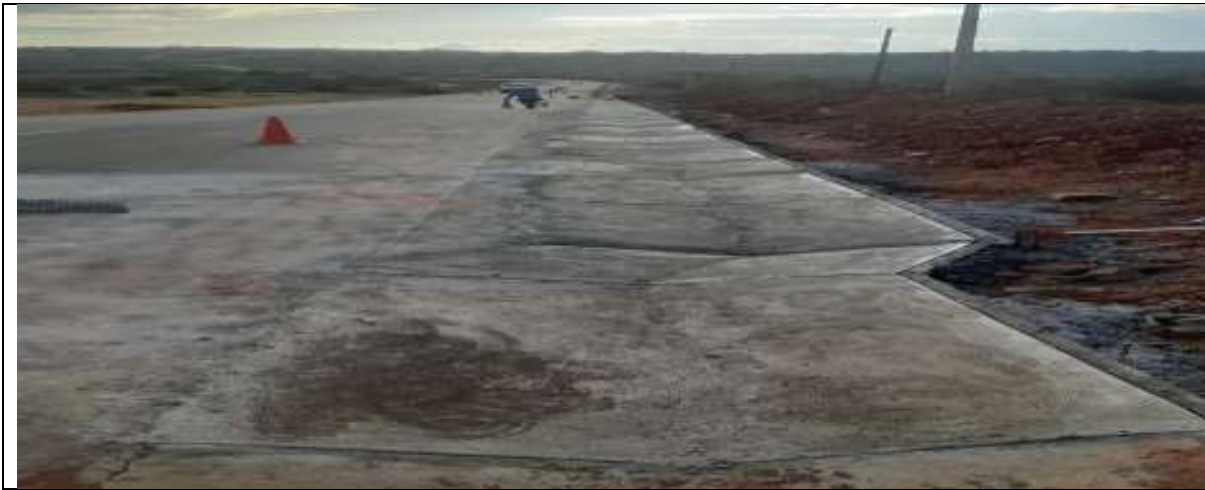
Upgrading of Arterial road in Ga Rampheri
