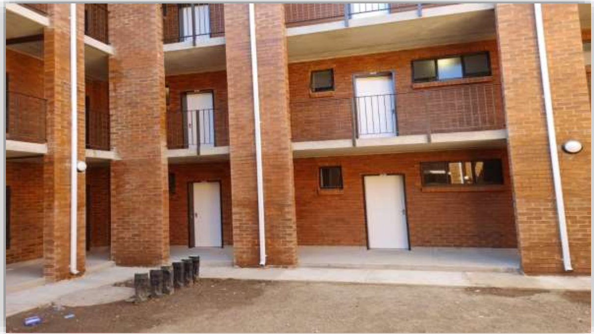
Ga-Rena Phase 2 Completed
