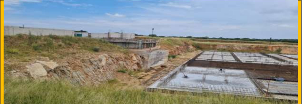
New Regional Wastewater Treatment Plant
