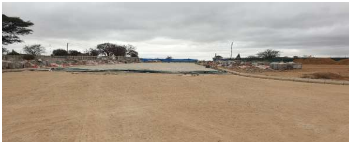
(Paving of internal Steets) at the Bus Depot at Seshego (1)
