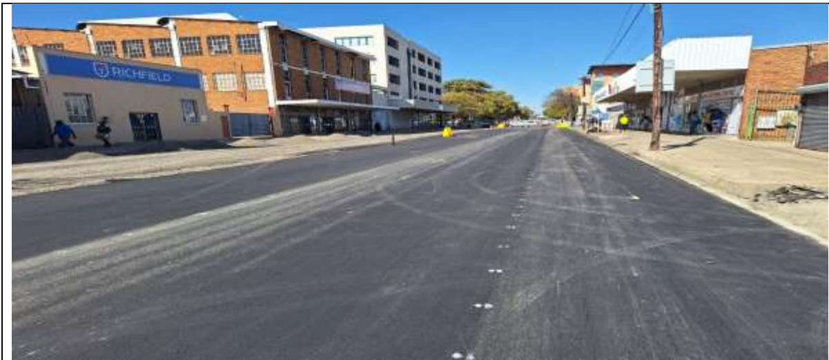
Rehabilitation of Church street ( City CBD )
