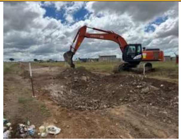
Upgrading of roads at Gamosi Via Chebeng to Sengatane ward 16
