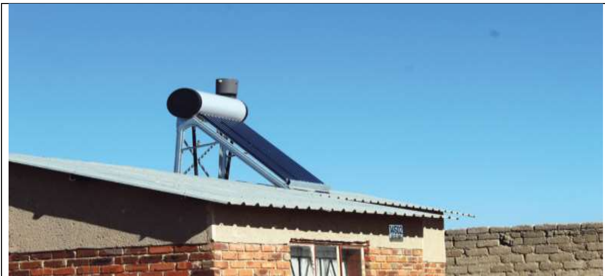
Solar geysers Installed at Seshego's Ext 71 and 75
