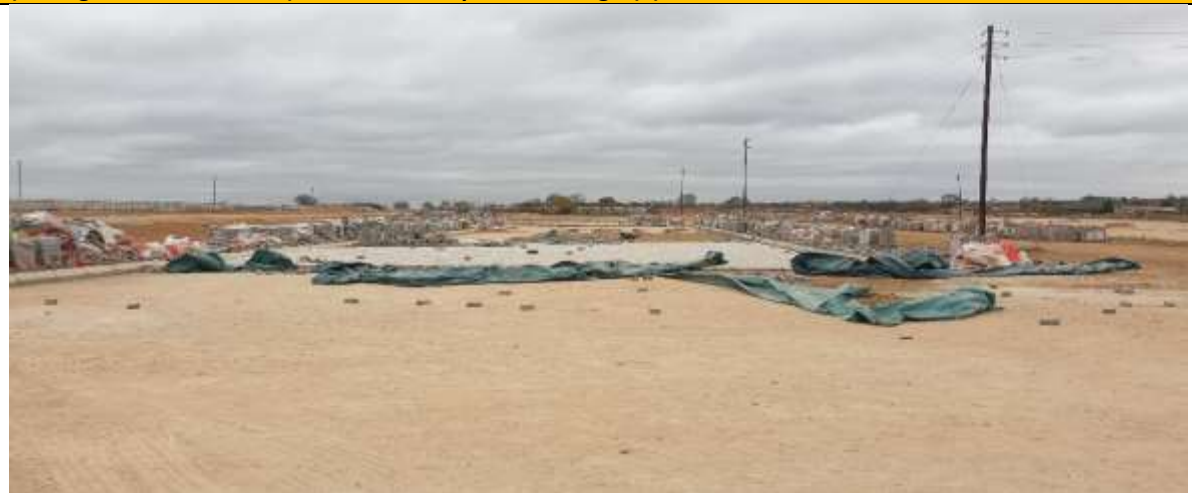
(Paving of internal Steets) at the Bus Depot at Seshego (2)
