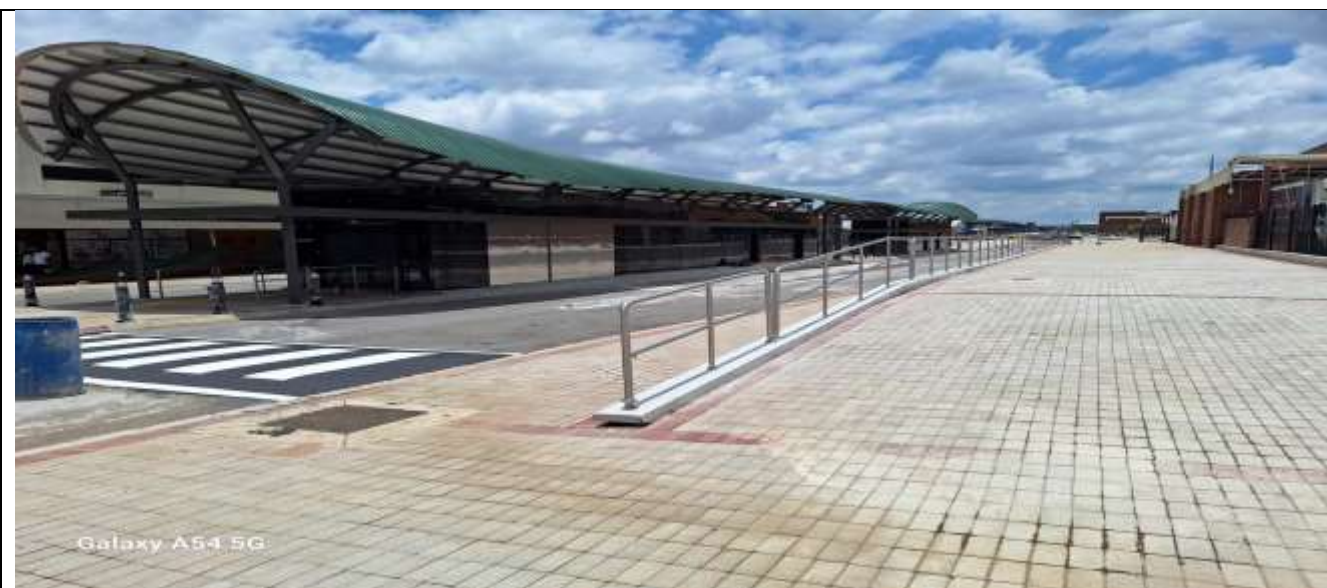
Construction of Leeto Bus Station at the City CBD (2)
