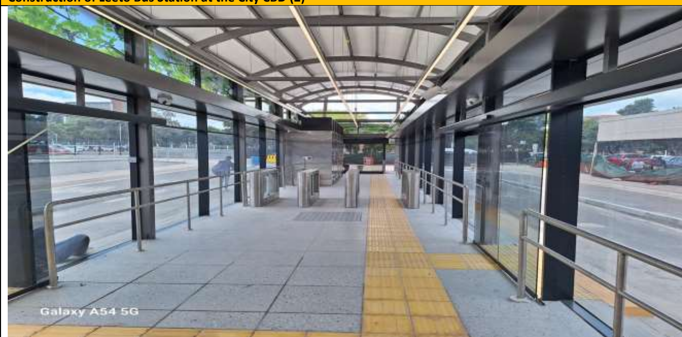
Construction of Leeto Bus Station at the City CBD (3)
