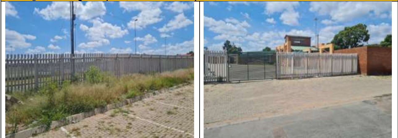
Fencing of Itsoseng Entrepreneurial Centre Completed 3
