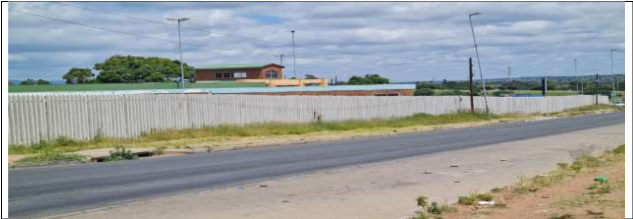
Fencing of Itsoseng Entrepreneurial Centre Completed 2
