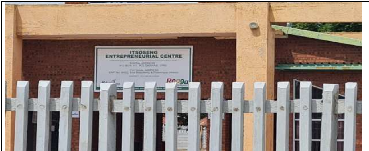
Fencing of Itsoseng Entrepreneurial Centre Completed 1
