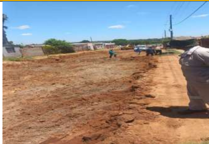
Upgrading of Roads in Westernburg ward 19
