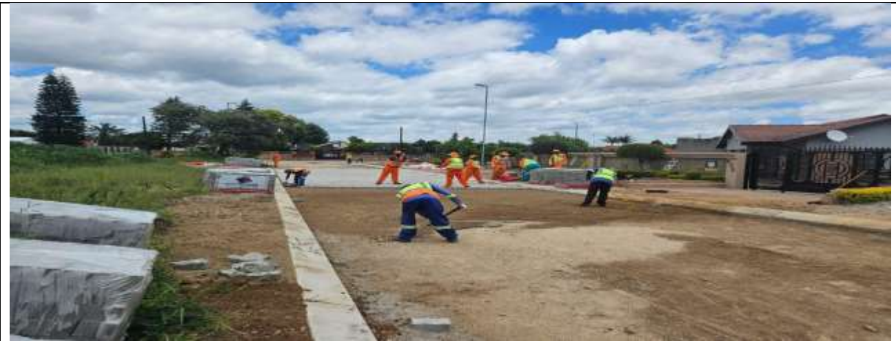
Paving of Economically Strategic Roads
