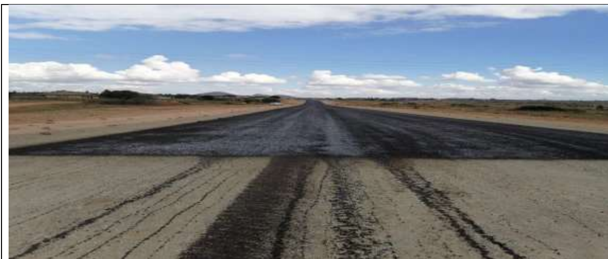
Upgrading of road from Mohlonong to Kalkspruit
