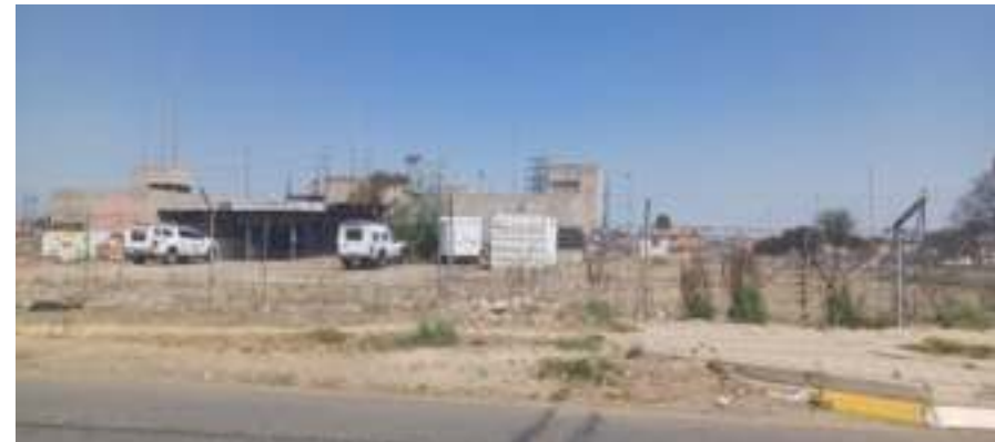
Diagram 176: Thornhill Substation to the south of the CBD
