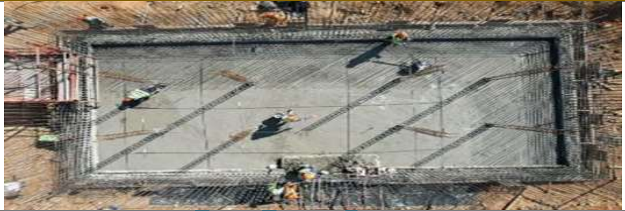
New Regional Wastewater Treatment Plant
