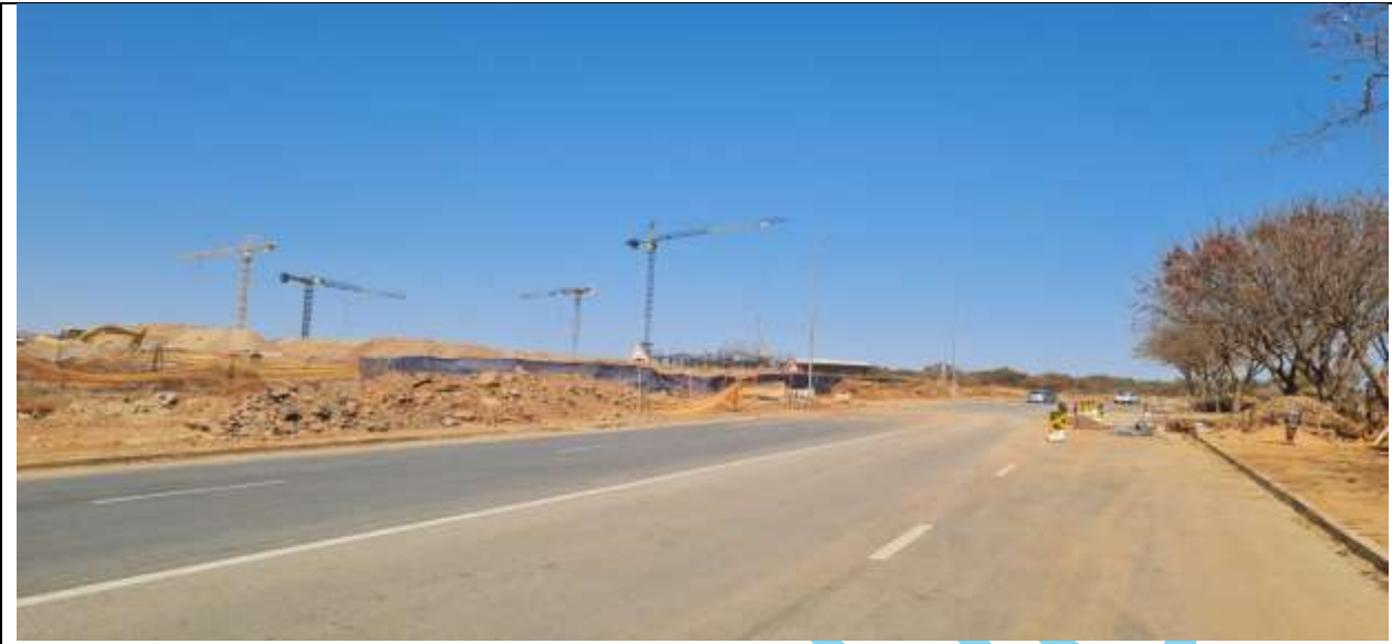
Construction of the New Limpopo Central Hospital
