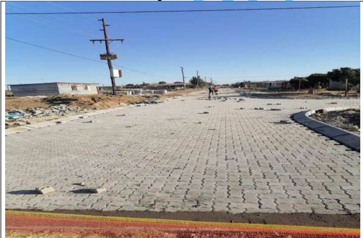
Paving of road at Extension 78
