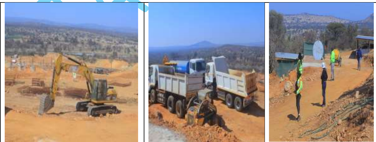
Construction of Limpopo Provincial Theatre (1)
