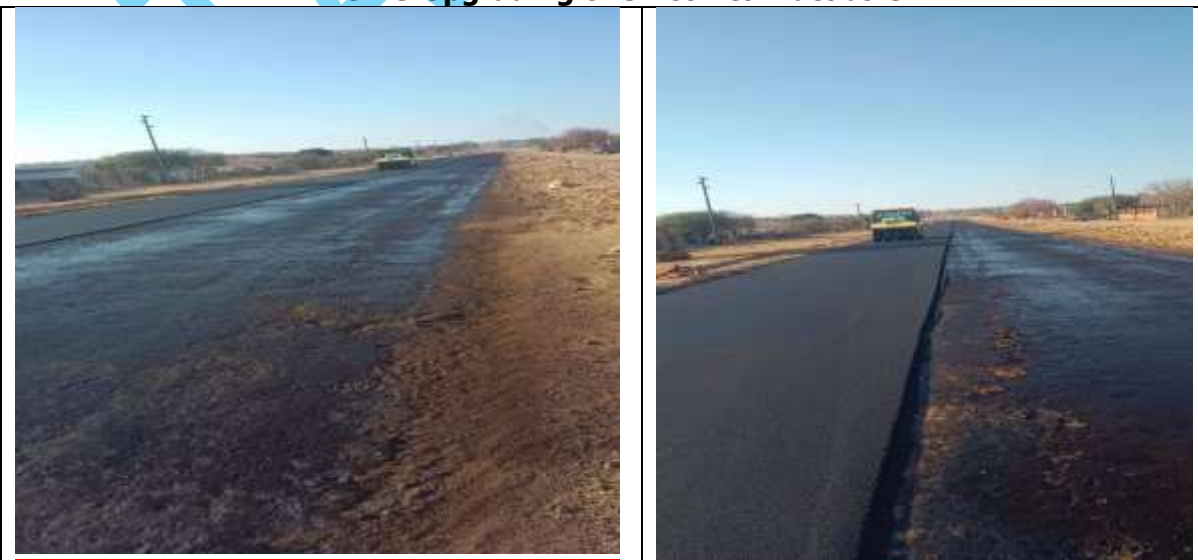
Upgrading of Silicon to Matobole
