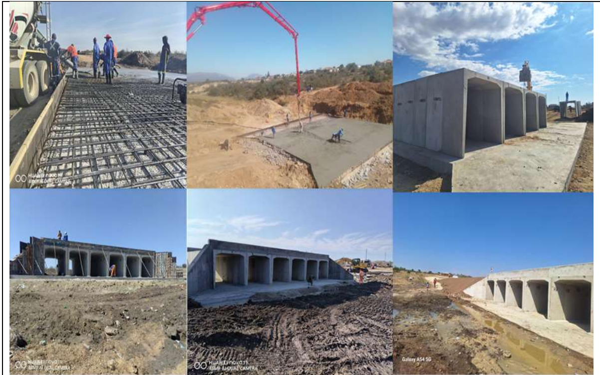
Low level bridges
