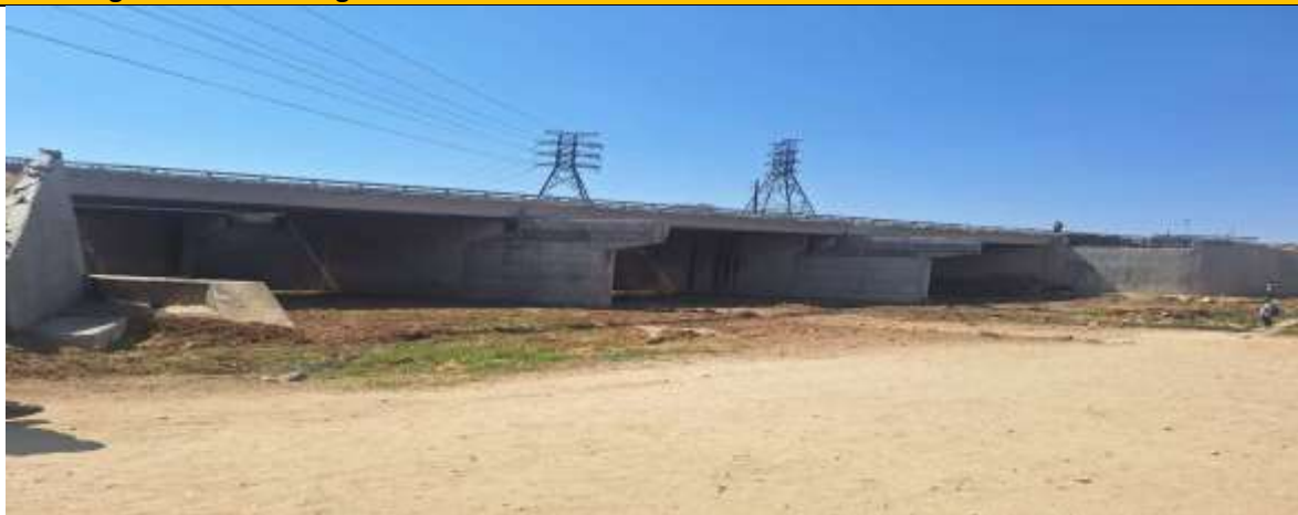
Widening of Sandriver Bridge 3
