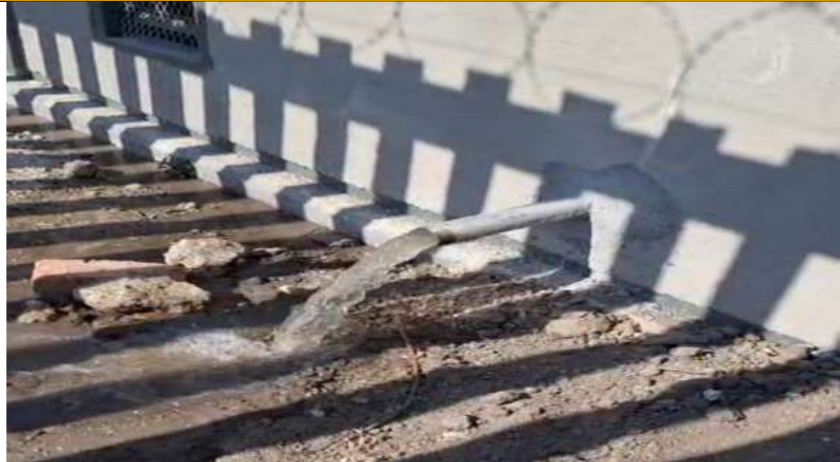
Sebayeng/Dikgale Regional Water Supply (RWS) Phase 10
