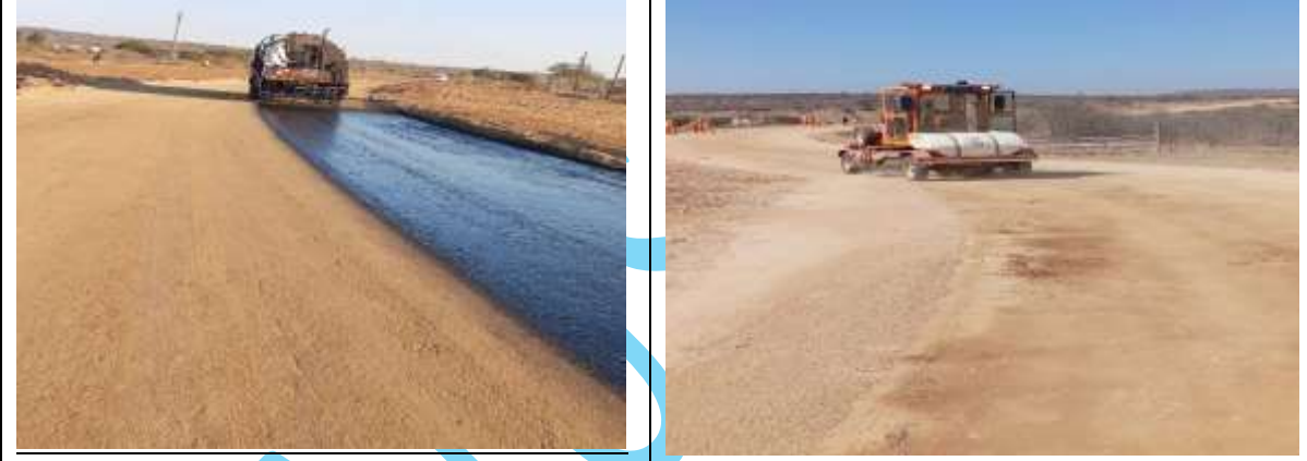
Upgrading of Access Road at Ga Makgoba (Ward 33)
