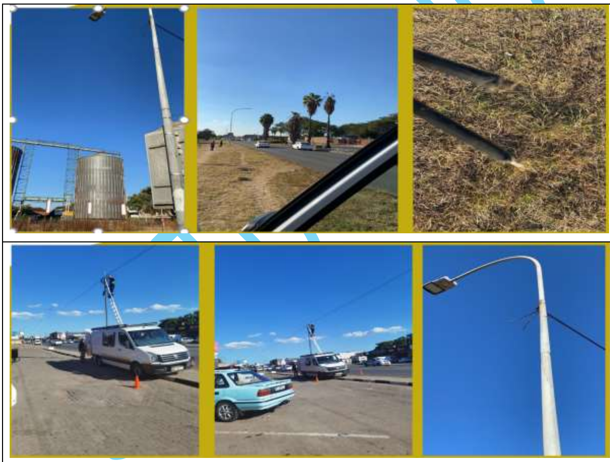
Figure: Damage and repair process of fibre connection.
