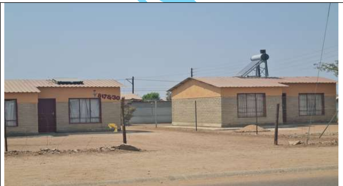
The two types of solar water geysers installed at Mohlakaneng Source: PLK Energy Services Directorate
