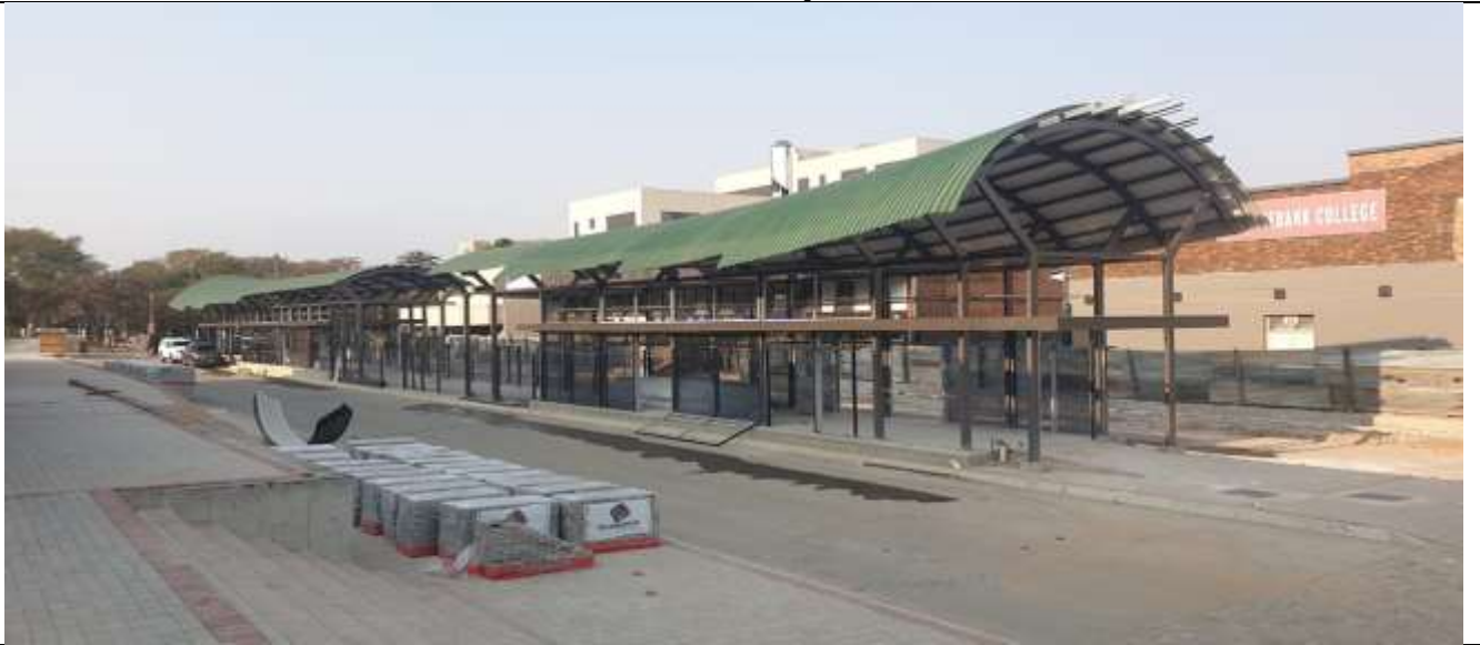
Construction of Leeto Bus Station at the City CBD (1)
