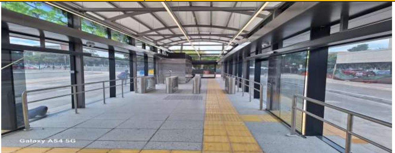
Construction of Leeto Bus Station at the City CBD (3)
