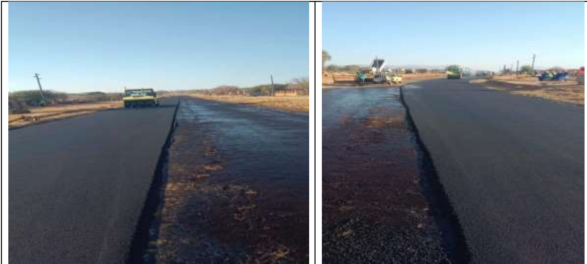
Upgrading of Silicon to Matobole
