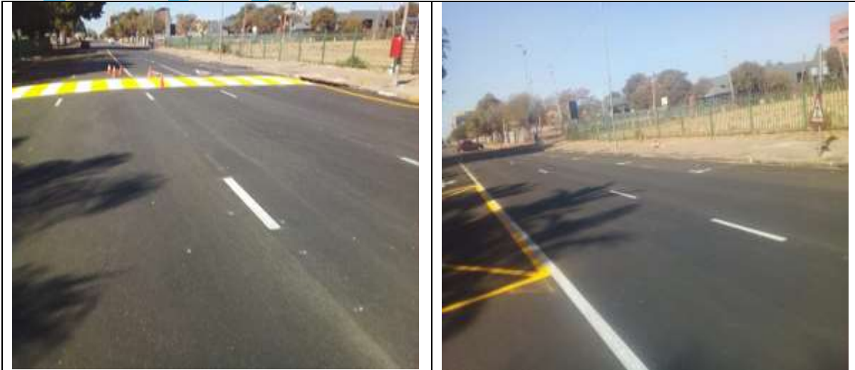
Road Marking at Bodenstein Street
