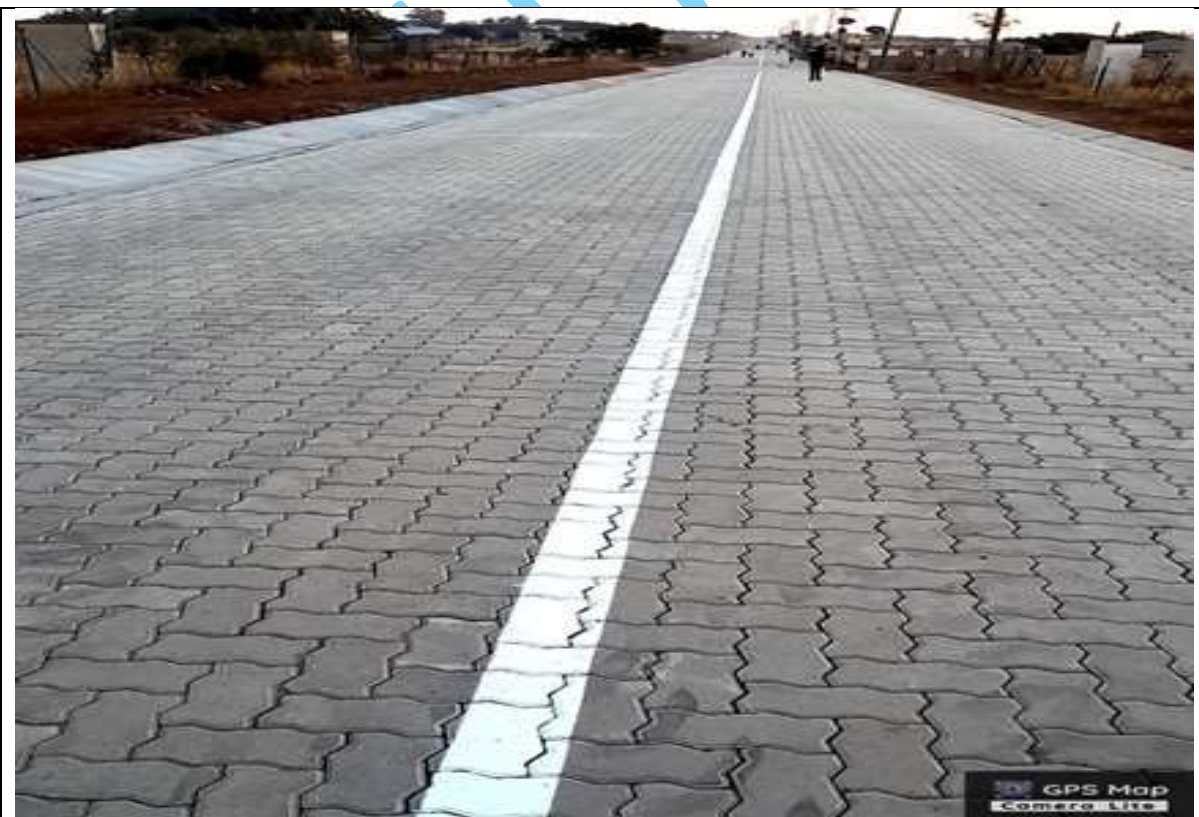
Paving of streets in Sebayeng /Dikgale cluster
