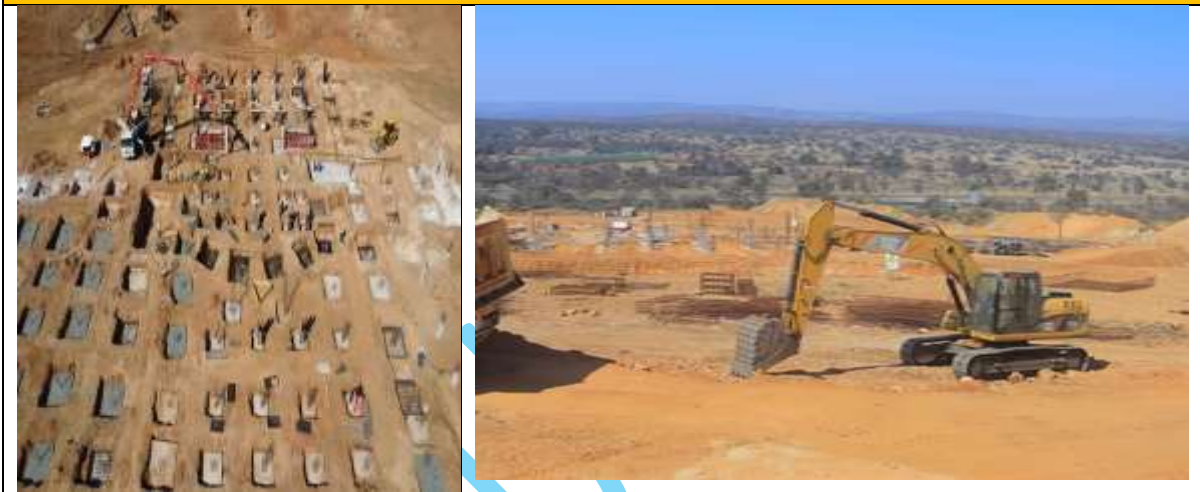
Construction of Limpopo Provincial Theatre(3)
