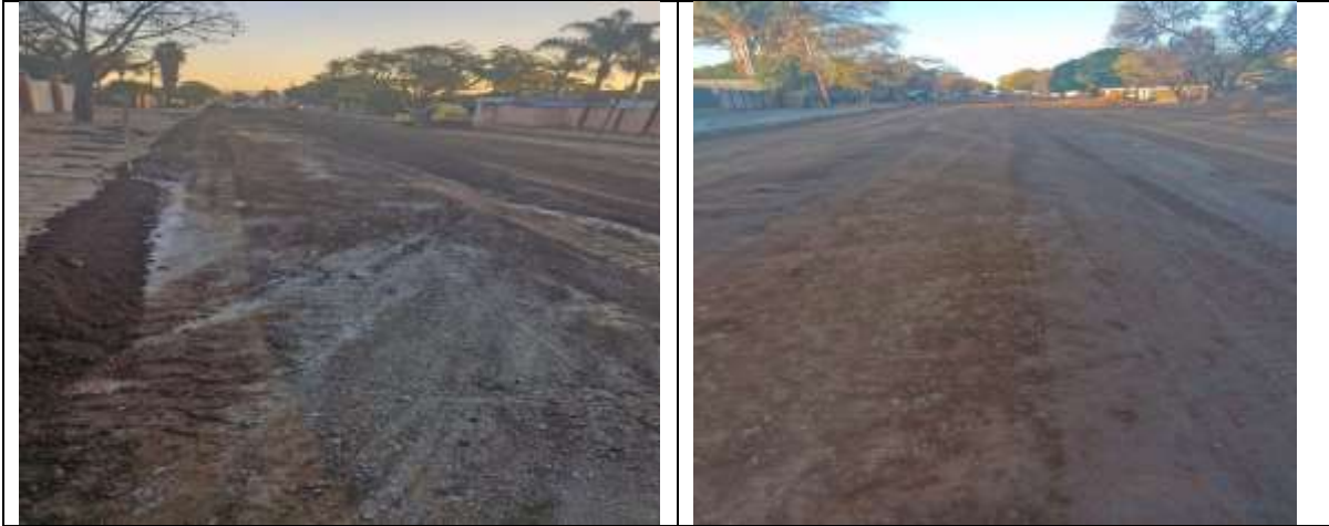
Rehabilitation of Jorrisen Street
