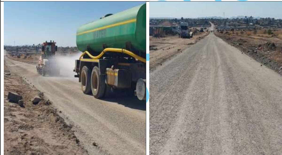
Upgrading the road from Ga-Mosi to Sengatane
