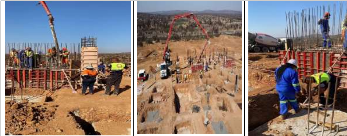
Construction of Limpopo Provincial Theatre(2)
