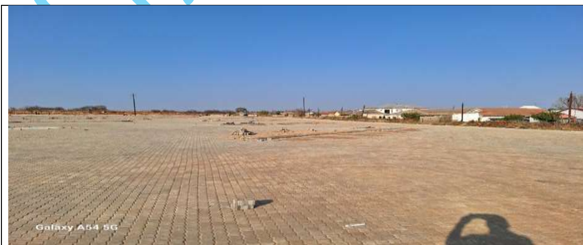
Paving of internal Streets at the Bus Depot at Seshego (2)
