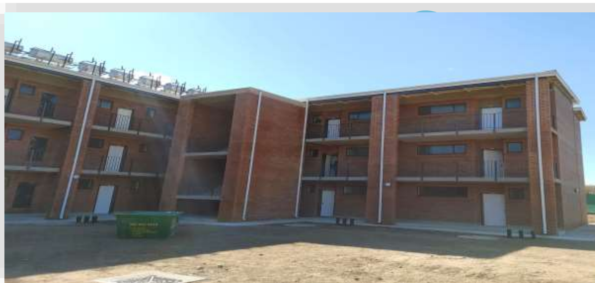
Annadale Ext 2 Completed
