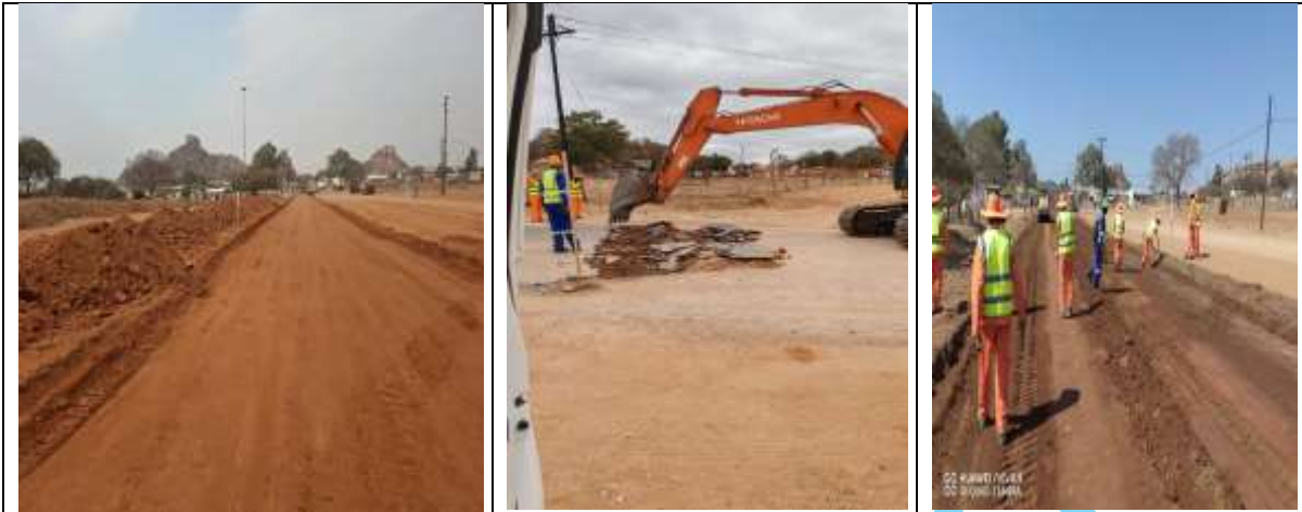
Paving of access road to Moshate wa Moletji (Offices )
