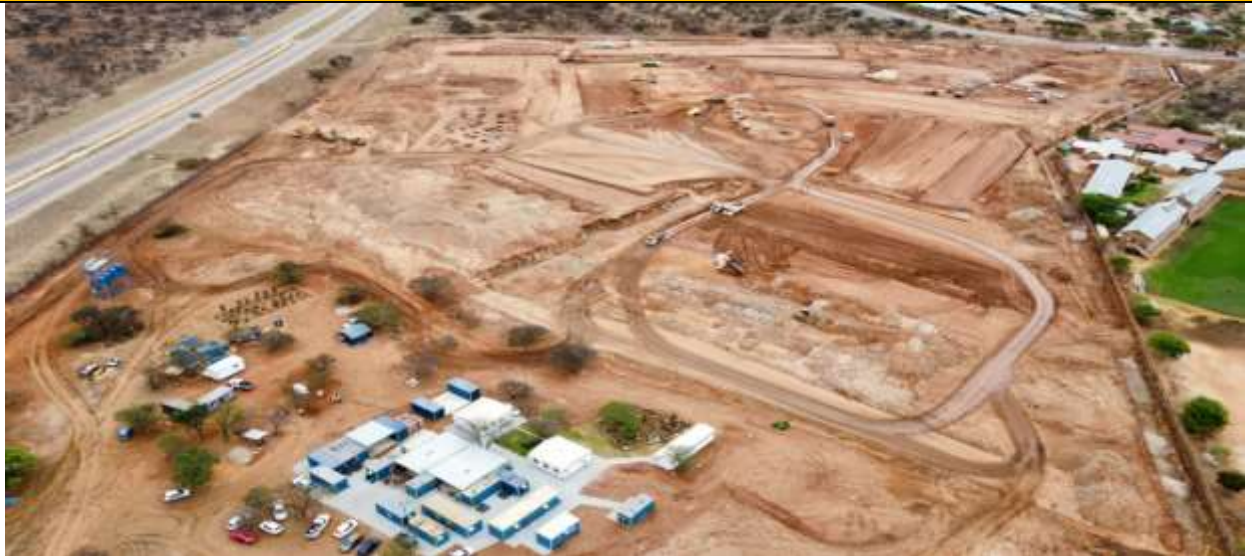
Bulk Underground Services Installation
