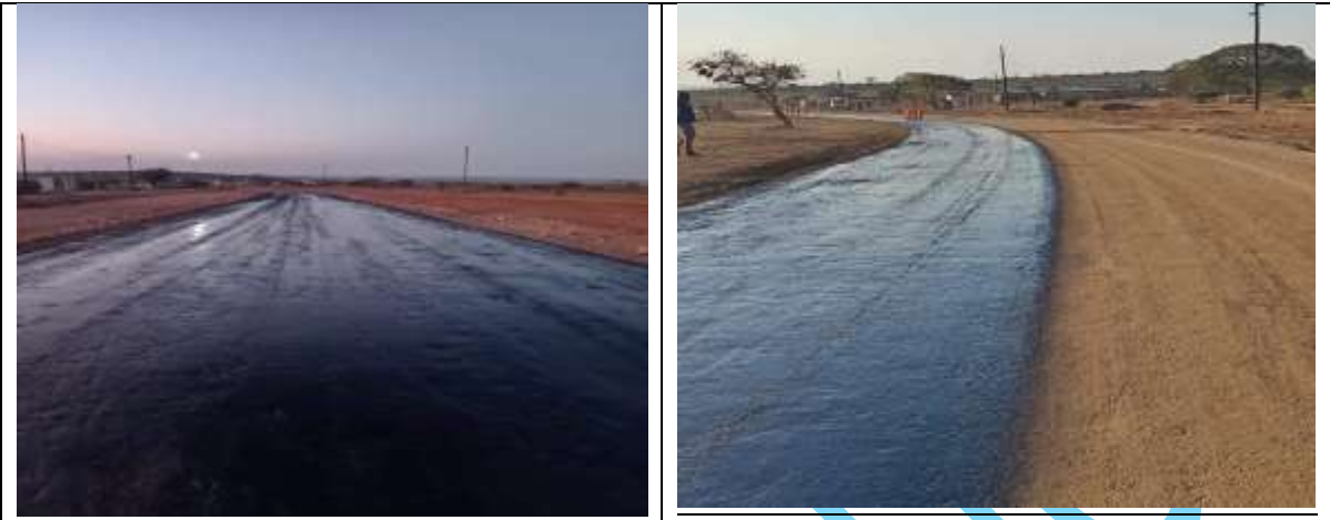
Upgrading of Access Road at Ga Makgoba (Ward 33)
