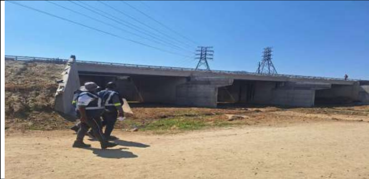
Widening of Sandriver Bridge 1
