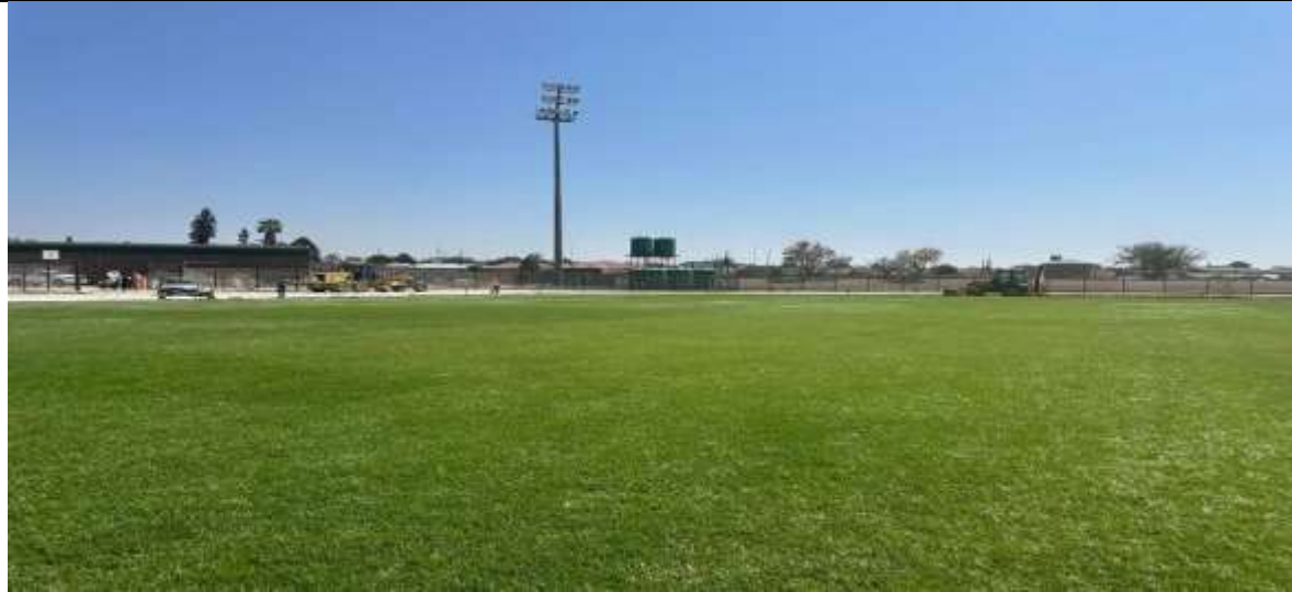
Completed Project -Upgrading of Seshego Stadium
