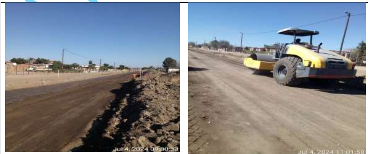
Upgrading of roads at Seshego Zone 6
