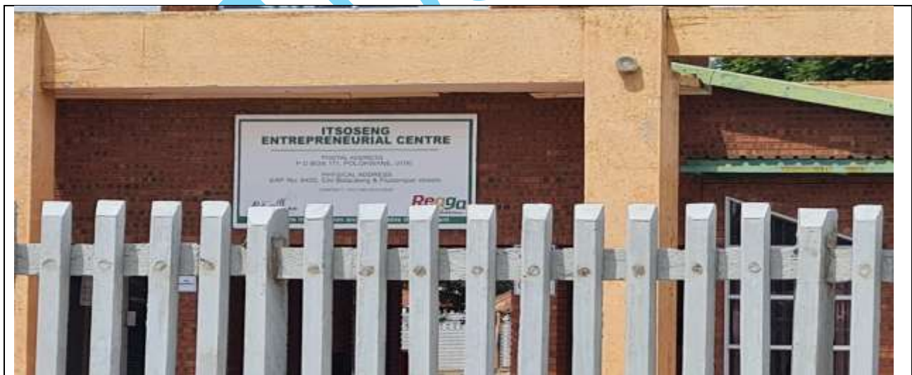
Fencing of Itsoseng Entrepreneurial Centre Completed 1
