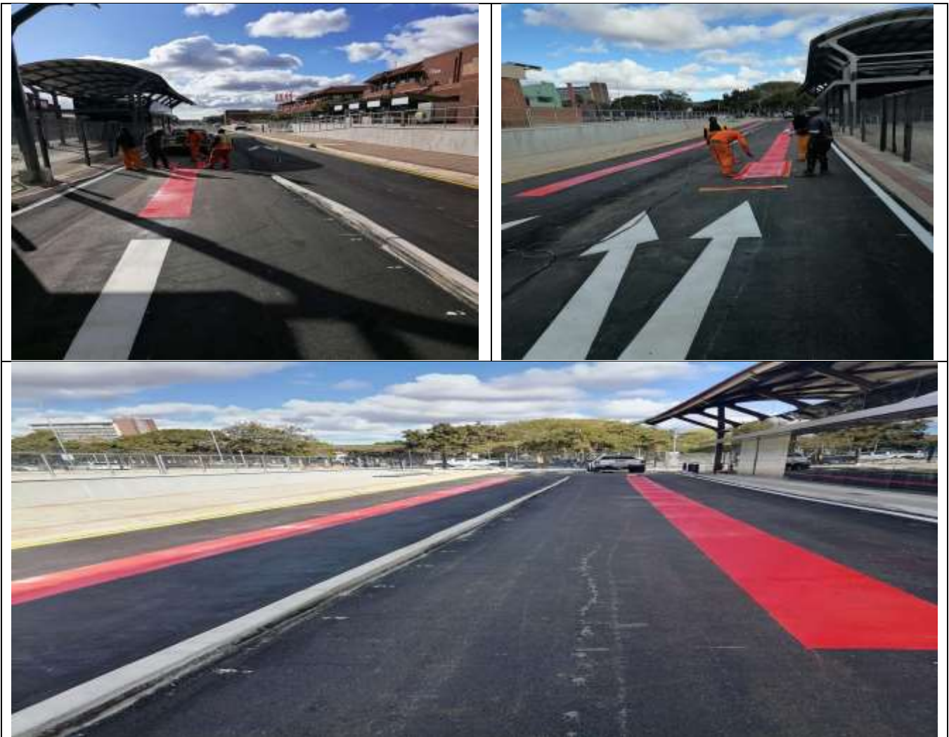
Construction of Leeto Bus Station at the City CBD (4)
