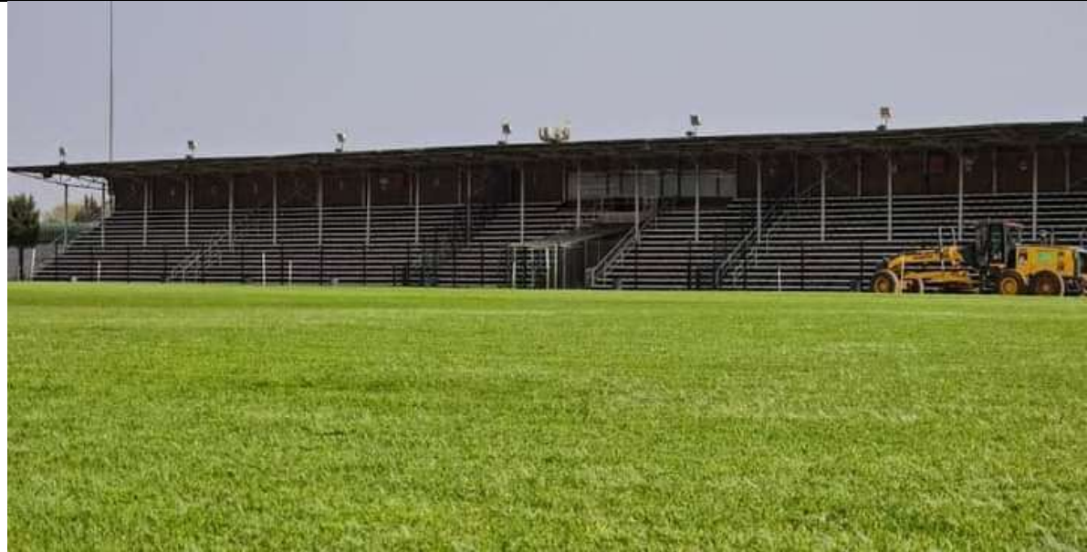
Completed Project -Upgrading of Seshego Stadium
