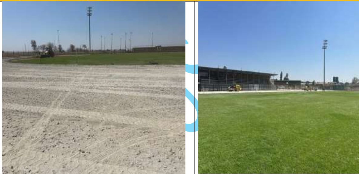
Completed Project -Upgrading of Seshego Stadium
