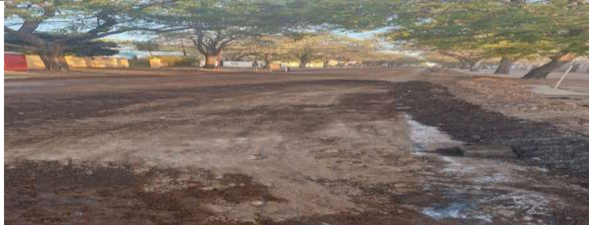
Rehabilitation of Jorrisen Street
