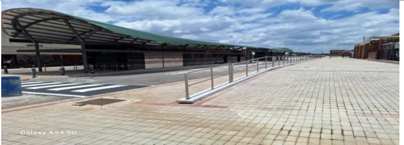
Construction of Leeto Bus Station at the City CBD (2)
