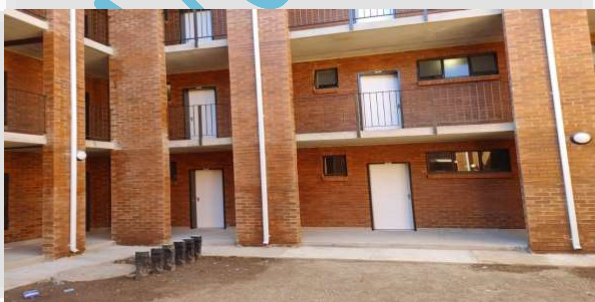
Annadale Ext 2 Completed
