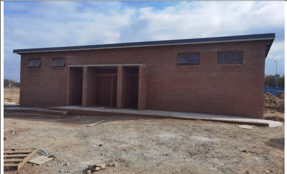
Completed Project - Construction of Ablution facility at Tom Naude Park
