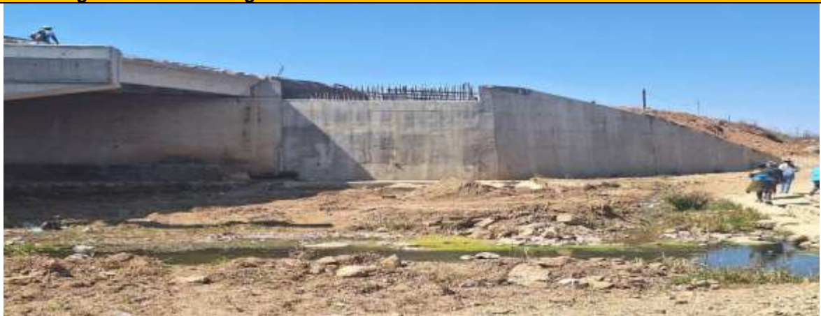
Widening of Sandriver Bridge 2
