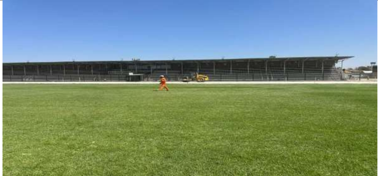
Completed Project -Upgrading of Seshego Stadium
