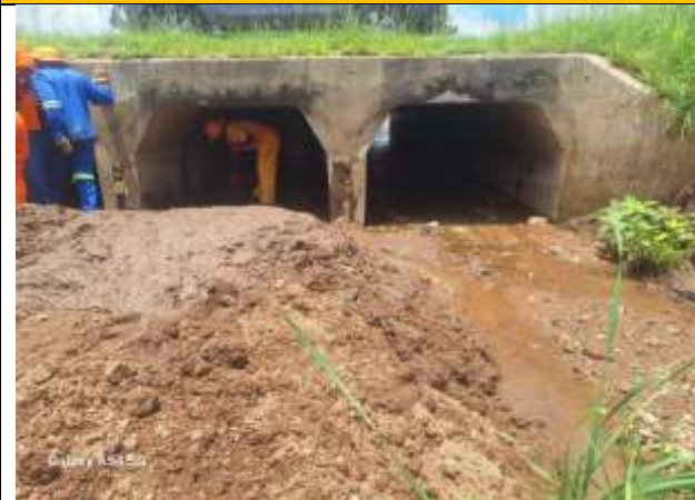
Unblocking Storm water Drainage System
