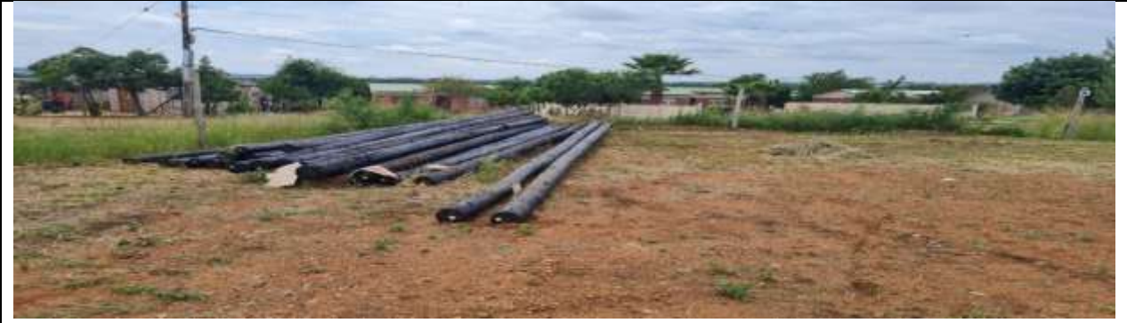
electrical network in Polokwane Ext 40, (146 households), including street lights
