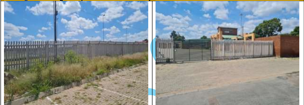
Fencing of Itsoseng Entrepreneurial Centre Completed 3
