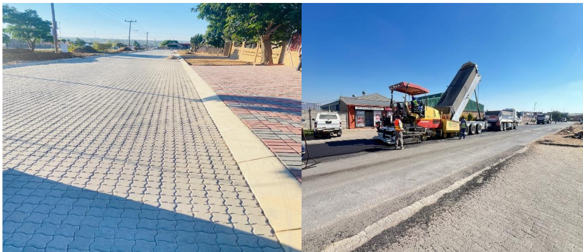
Paving of Internal streets in Seshego Zone 4
