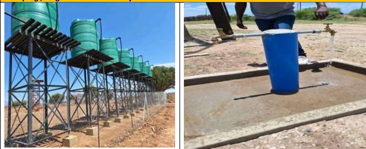
Sebayeng /Dikgale RWS water Project at Ward 31
