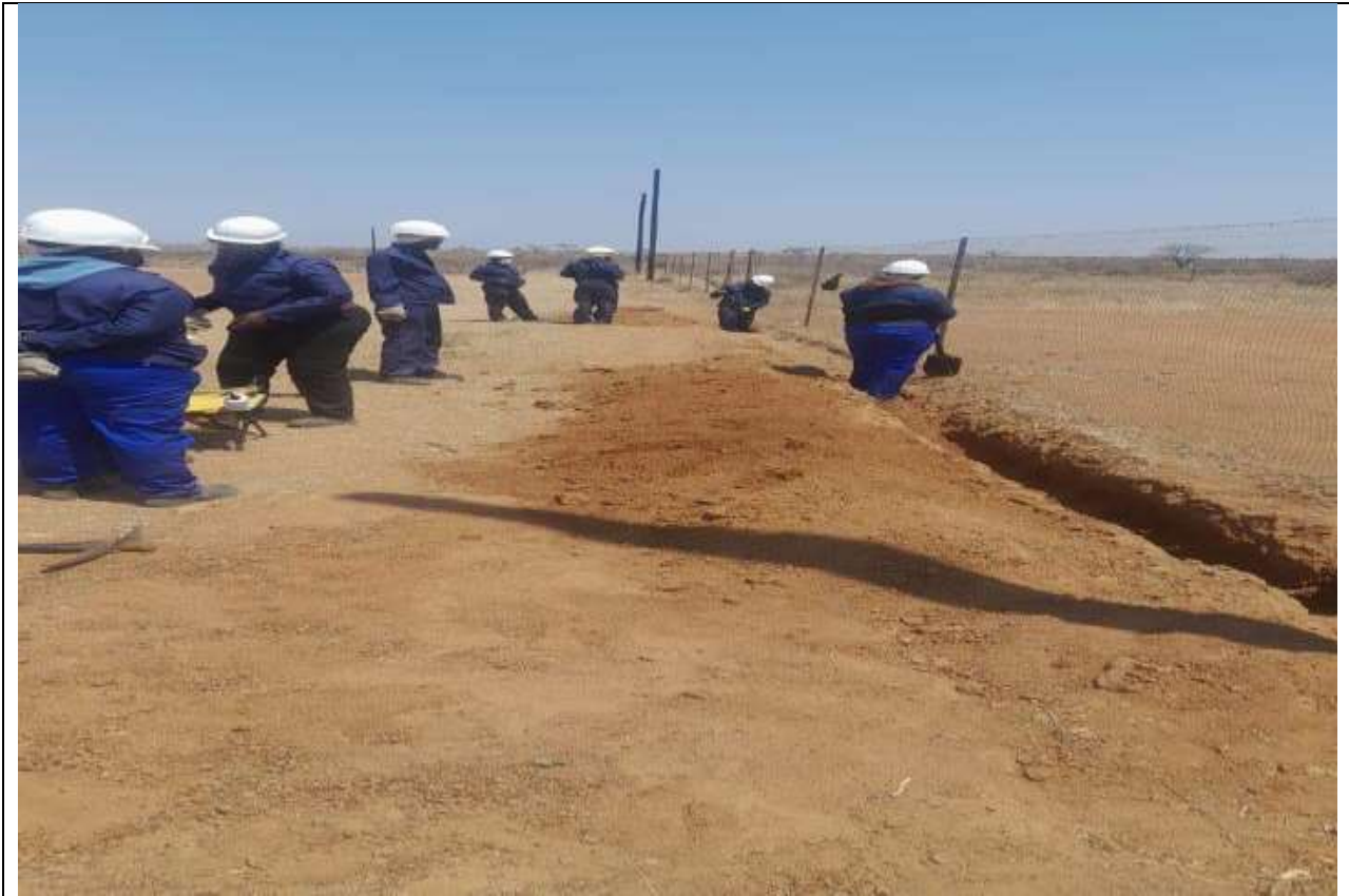
Electrification of Rammetloana Village in Ward 45
