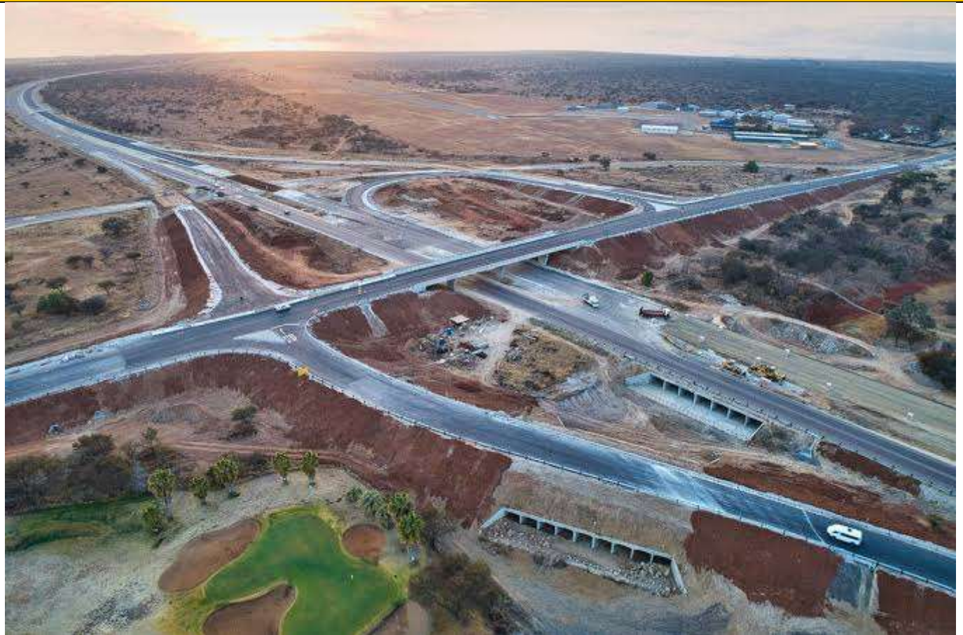
Polokwane Eastern Ring Roads – N1 bypass Next to Peter Mokaba Stadium
