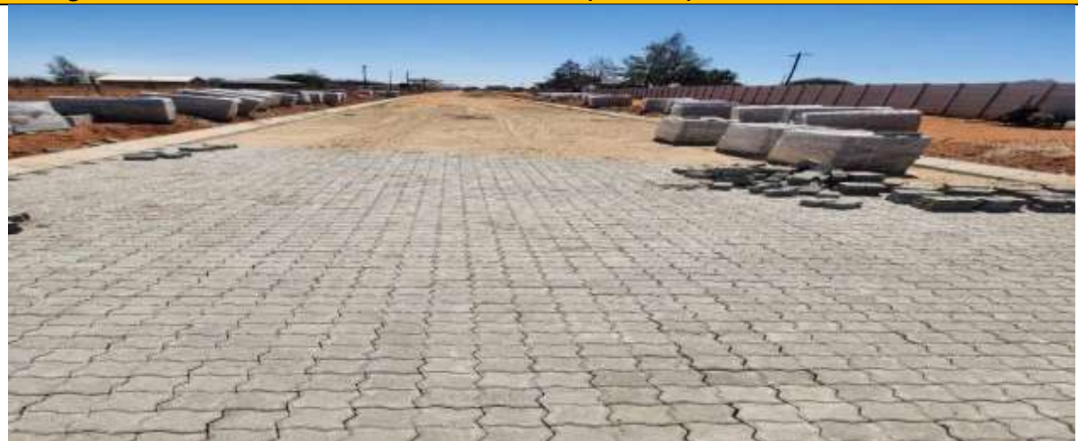
Paving of Internal Street from Solomondale to D3997(Ward 32)
