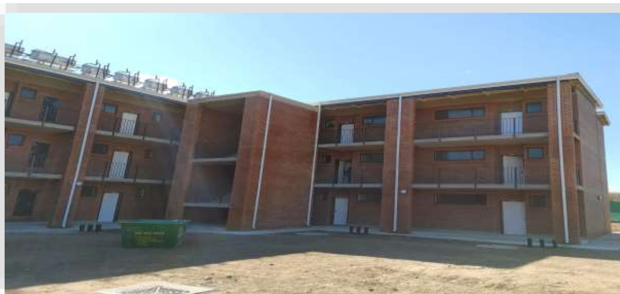
Annadale Ext 2 Completed
