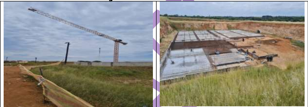
New Regional Wastewater Treatment Plant
