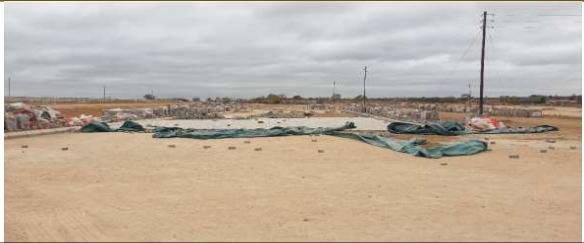
Paving of internal Streets at the Bus Depot at Seshego (2)
