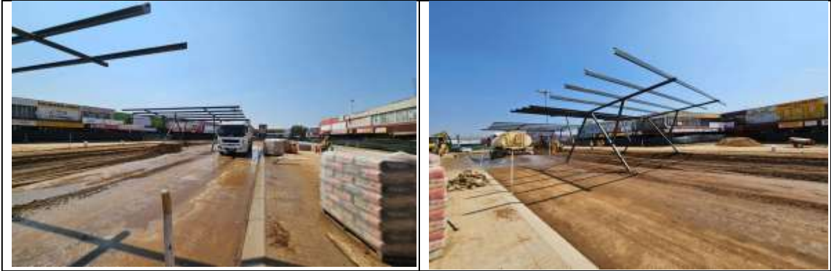
Shades Structures installed at Indian Centre Taxi Rank(2)
