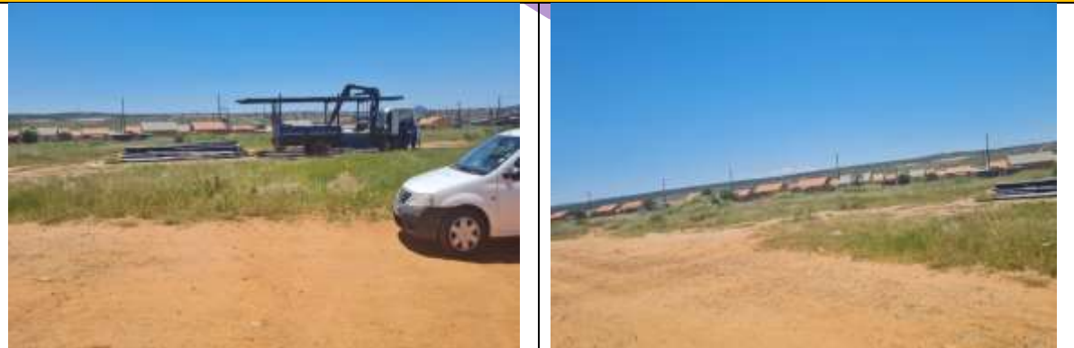
Electrification of Urban Households in Seshego Zone 8 Ext. 133 Phase 3.
