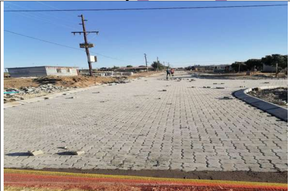
Paving of road at Extension 78
