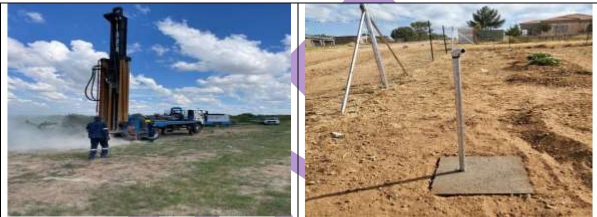
Kalkspruit/Mangongoa Water Supply Project
