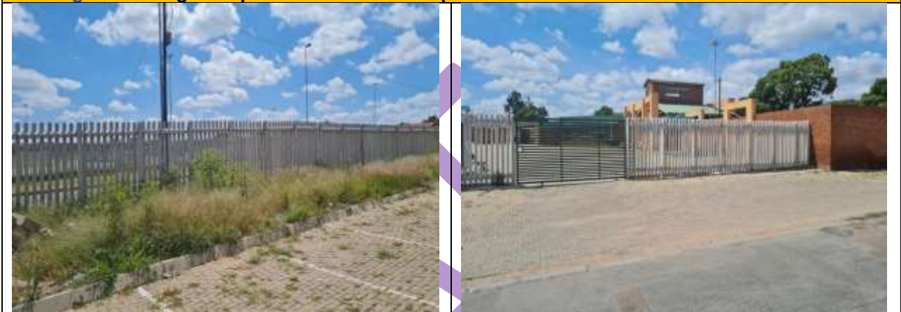
Fencing of Itsoseng Entrepreneurial Centre Completed 3
