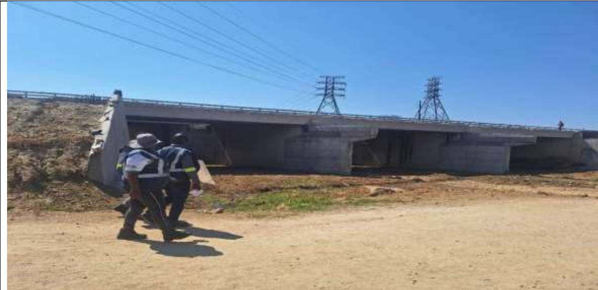
Widening of Sandriver Bridge 1
