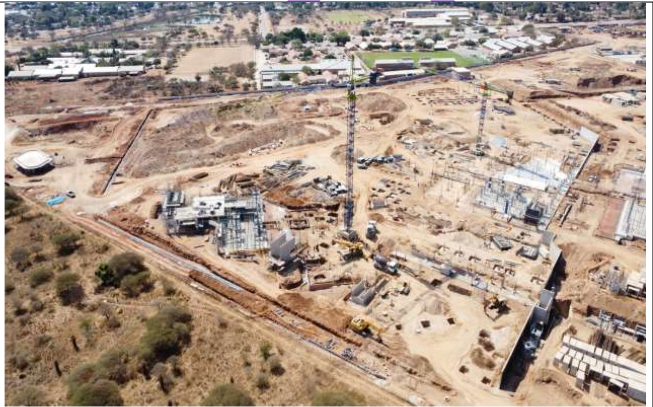
Construction of the New Limpopo Central Hospital
