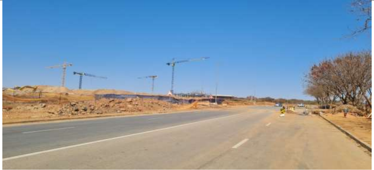
Construction of the New Limpopo Central Hospital
