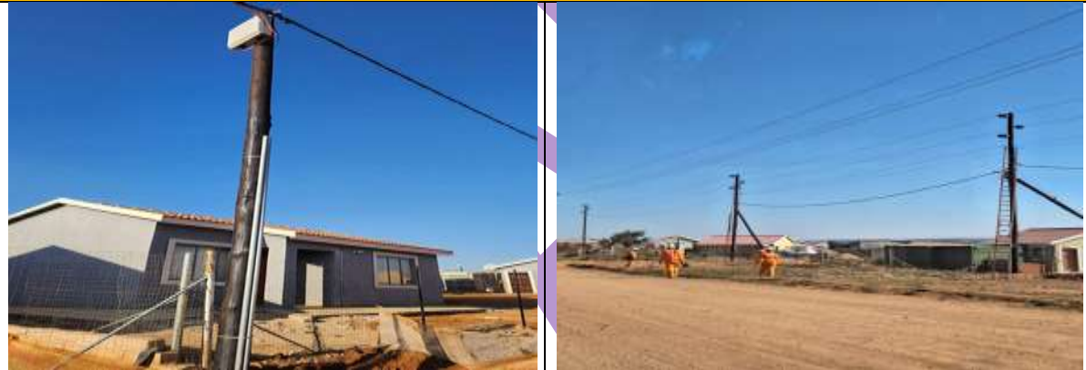
installation of electrical network in Polokwane Ext 40.
