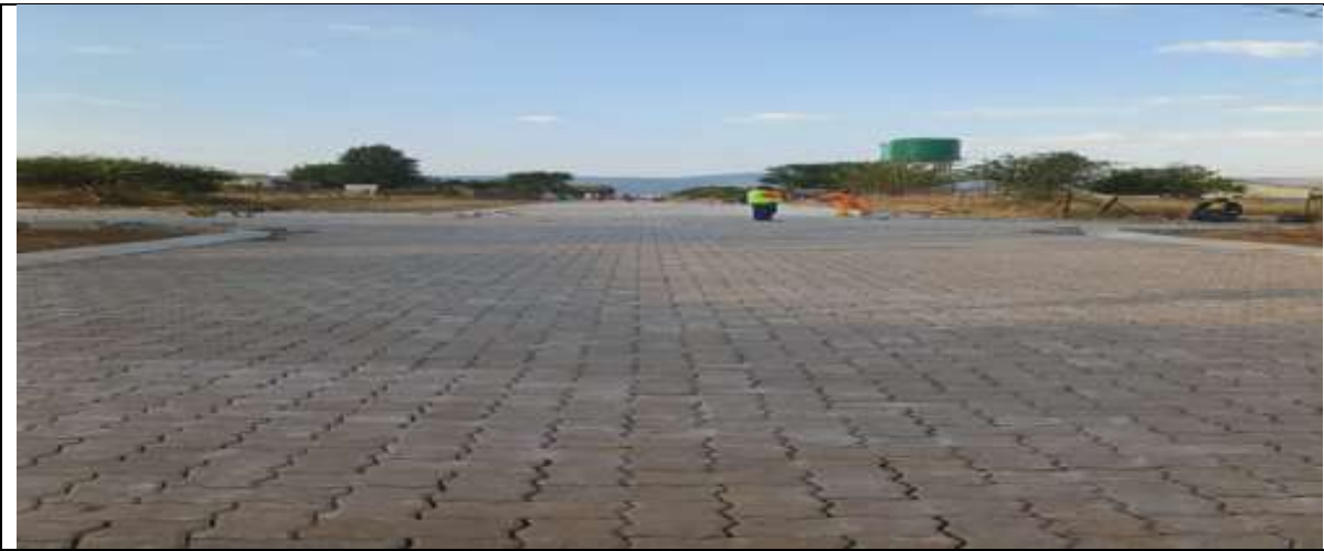
Paving of streets in Mankgaile
