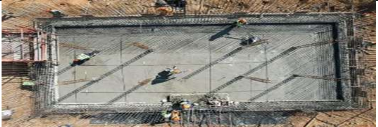
New Regional Wastewater Treatment Plant
