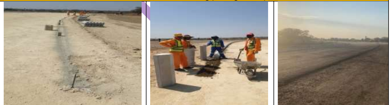
Construction of Nelson Mandela Bo-okelo, Ditlou Crossing (Seshego Circle)
