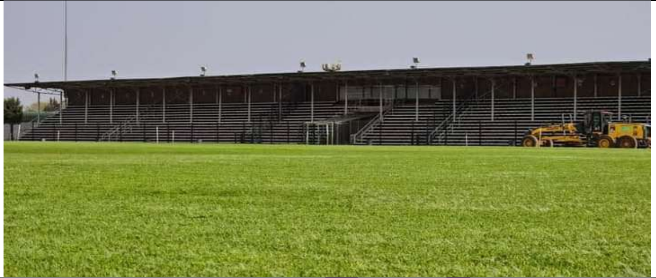
Completed Project -Upgrading of Seshego Stadium
