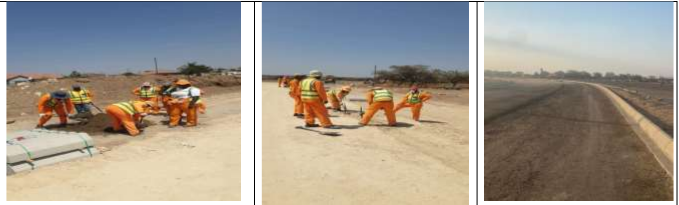
Construction of Nelson Mandela Bo-okelo, Ditlou Crossing (Seshego Circle)
