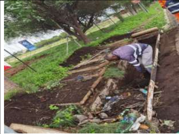
Unblocking Storm water Drainage System
