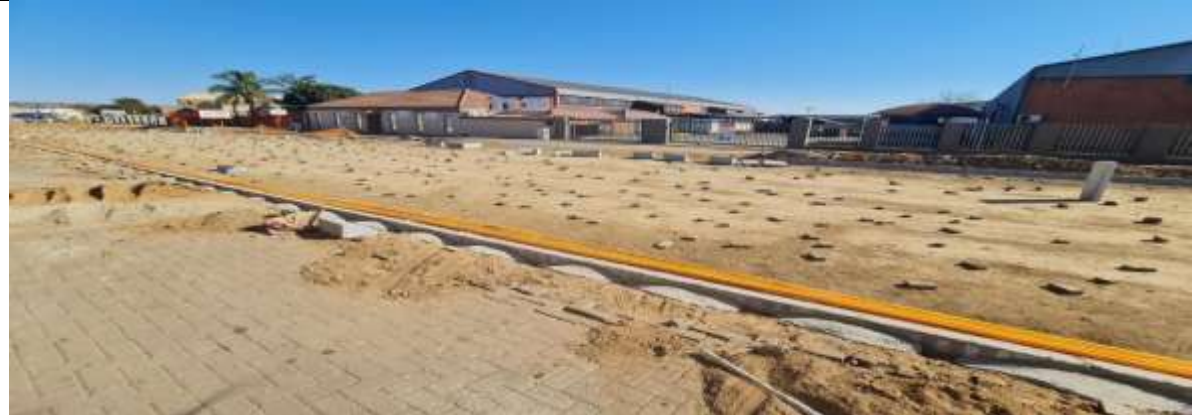
Rehabilitation of Blaauberg street between Bulawayo and fluorspar street (Industrial Area)
