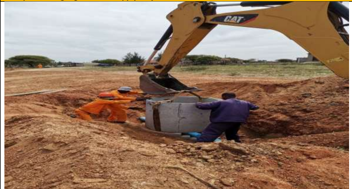
Kalkspruit/Mangongoa Water Supply Project
