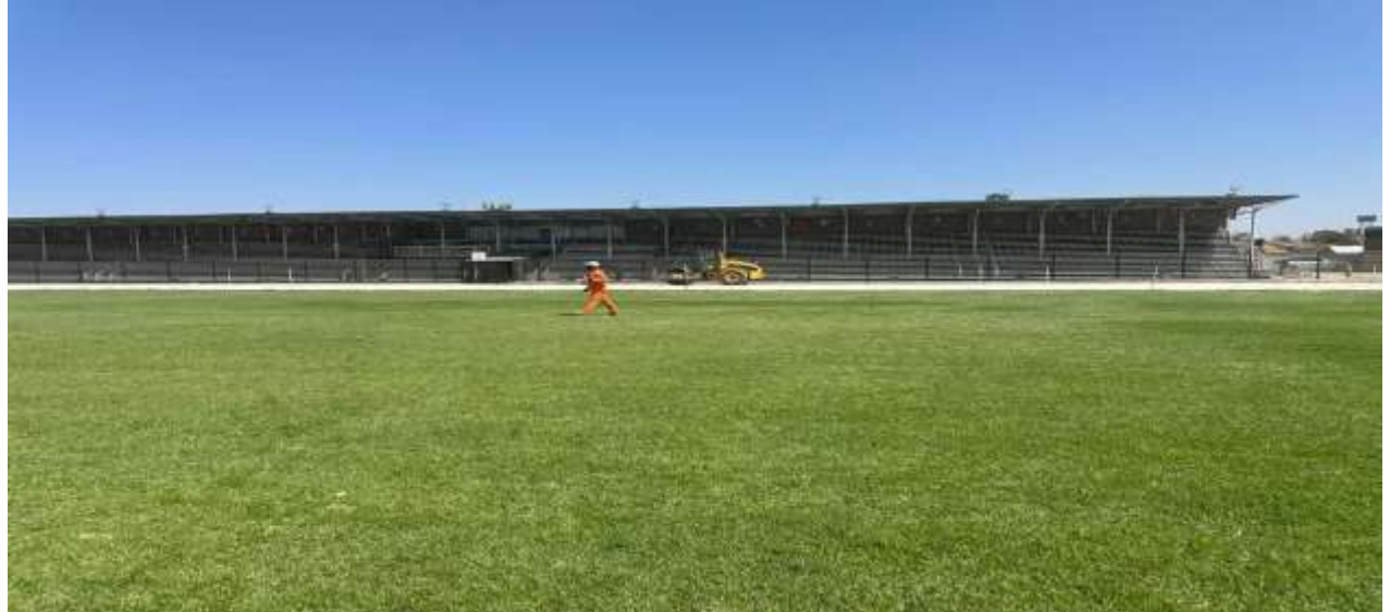
Completed Project -Upgrading of Seshego Stadium
