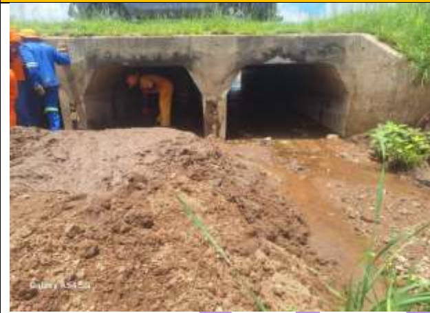
Unblocking Storm water Drainage System
