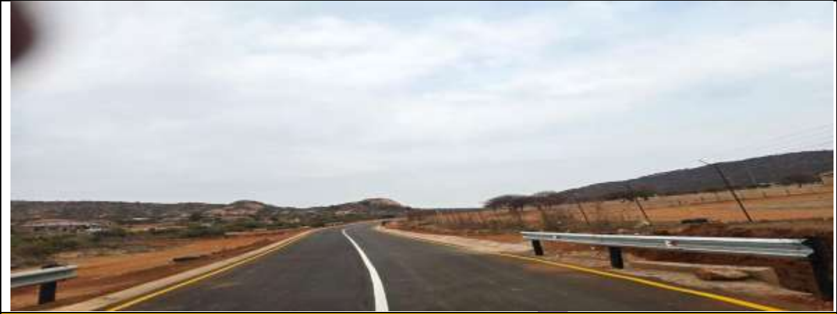
Upgrading of internal streets in Mountain view (3)
