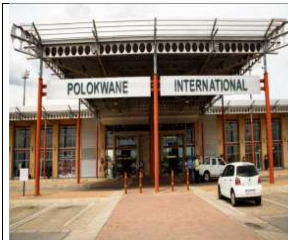
Polokwane International Airport 1
