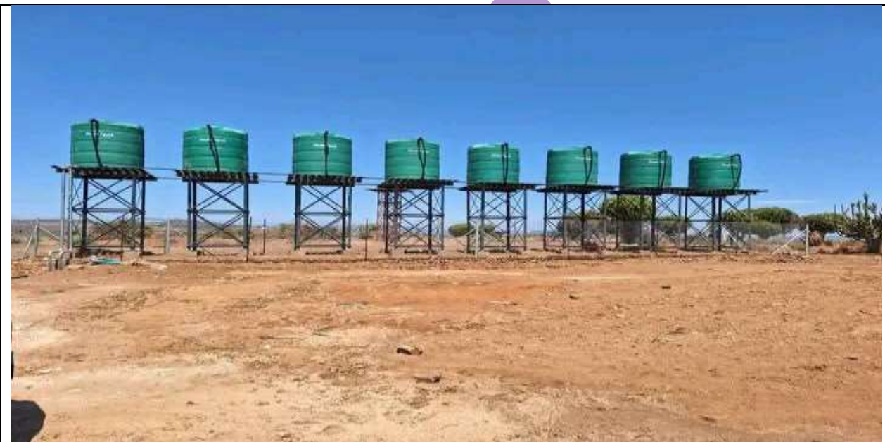
Sebayeng /Dikgale RWS water Project at Ward 31
