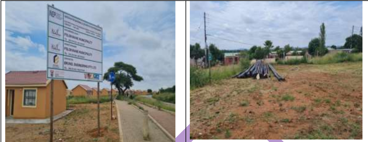
installation of electrical network in Polokwane Ext 40.
