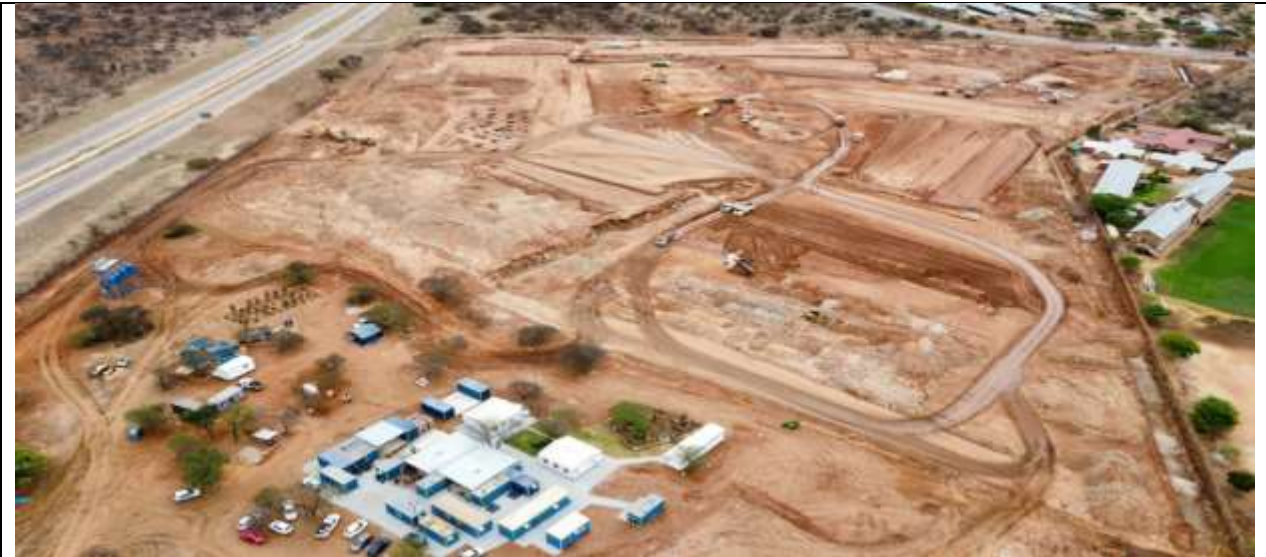
Bulk Underground Services Installation
