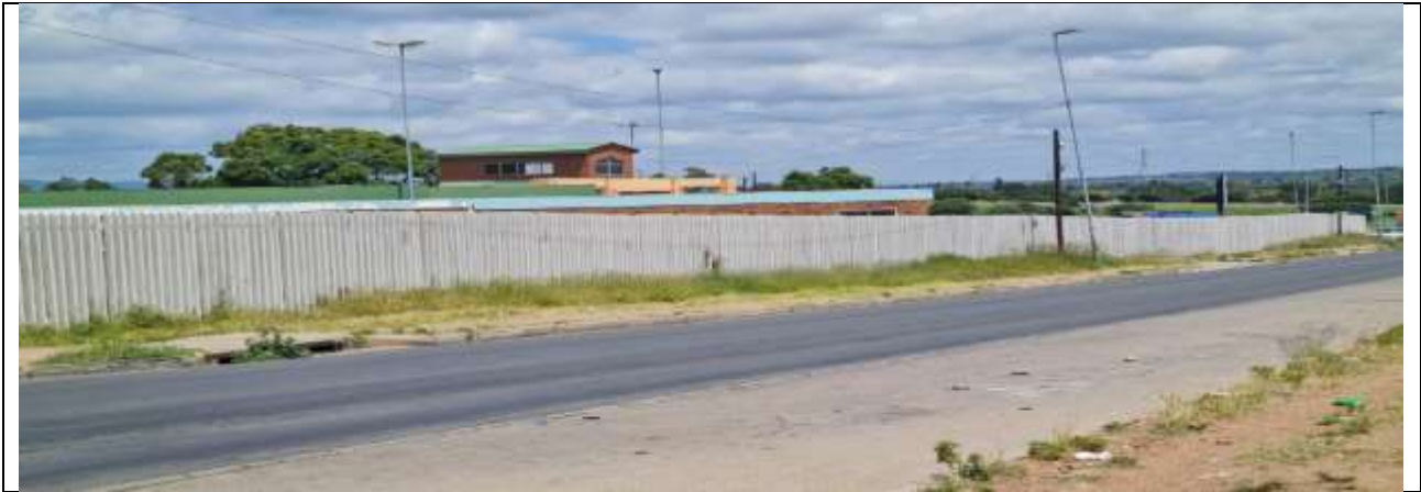
Fencing of Itsoseng Entrepreneurial Centre Completed 2
