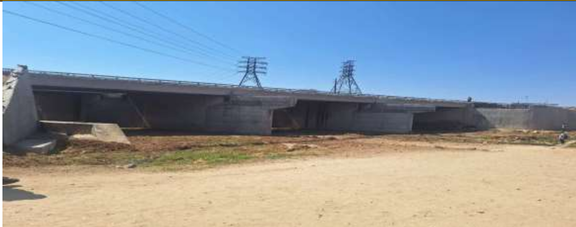
Widening of Sandriver Bridge 3
