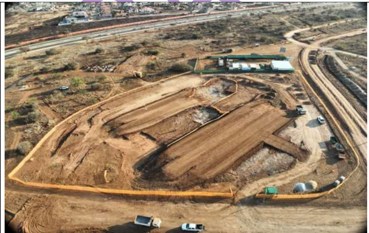
Construction of New NETCARE AKESO Psychiatric Hospital
