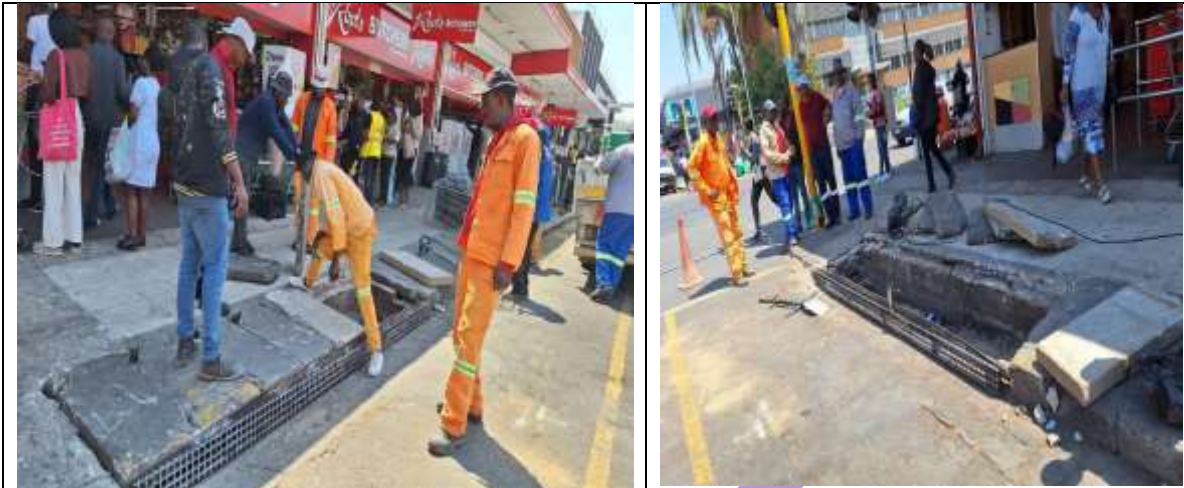
Unblocking of Storm Water Drainage System in the City CBD
