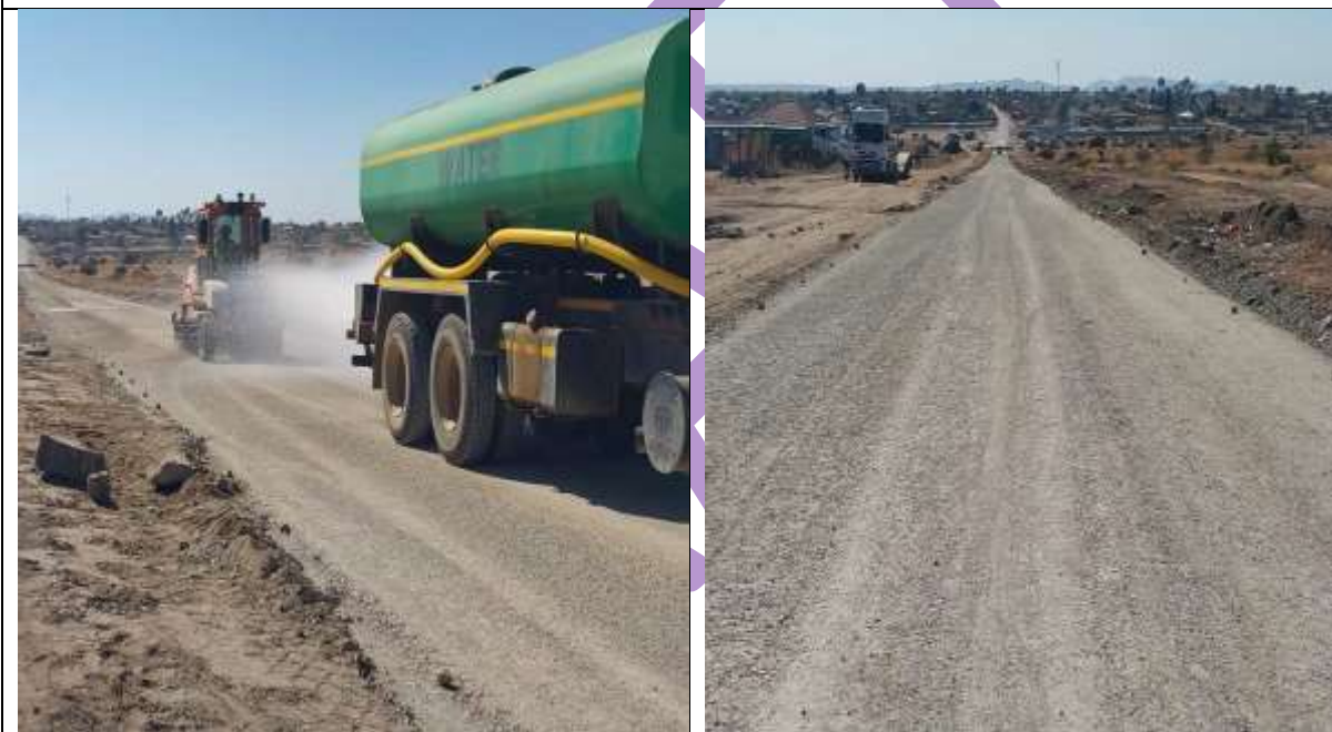
Upgrading the road from Ga-Mosi to Sengatane
