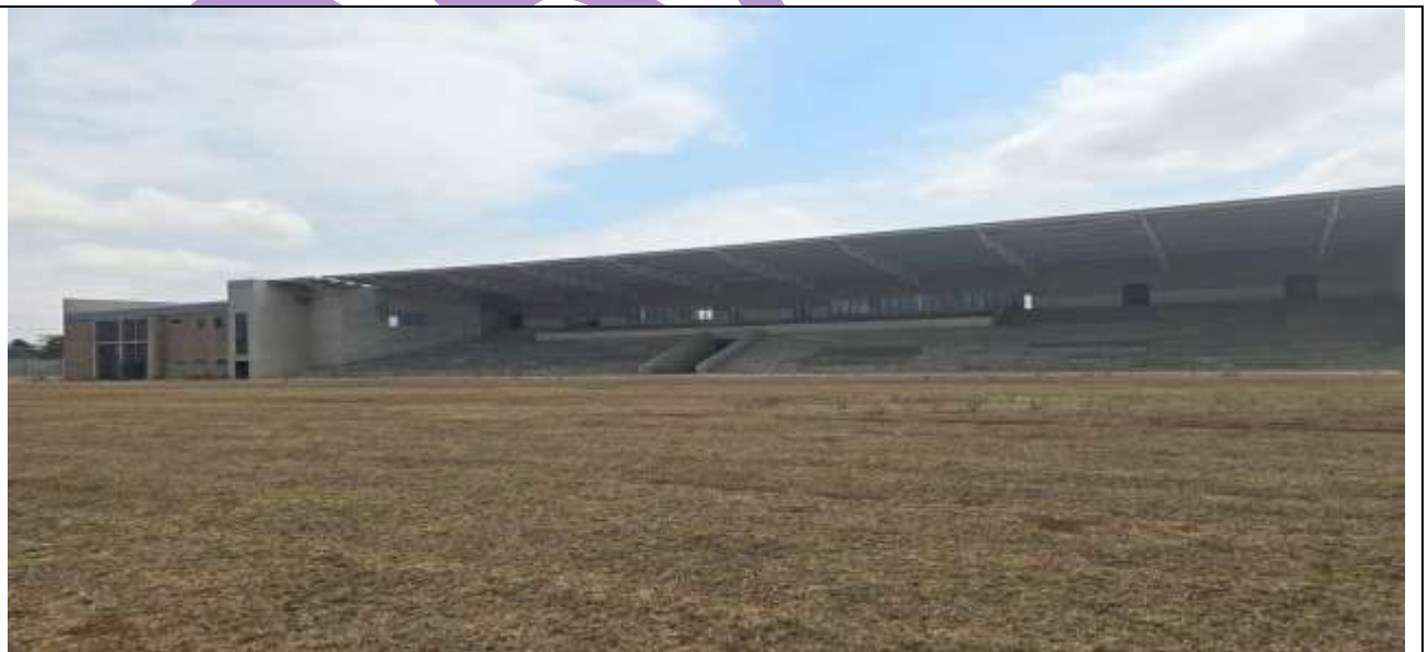
Construction of Mankweng Stadium
