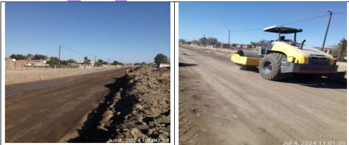
Upgrading of roads at Seshego Zone 6
