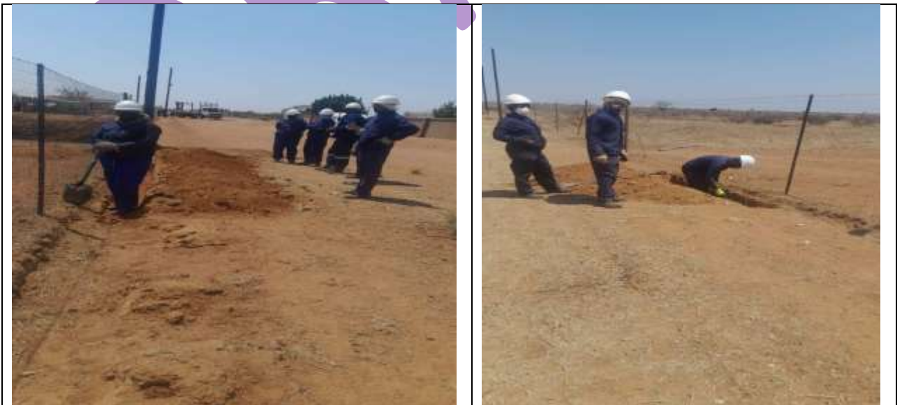
Electrification of Rammetloana Village in Ward 45
