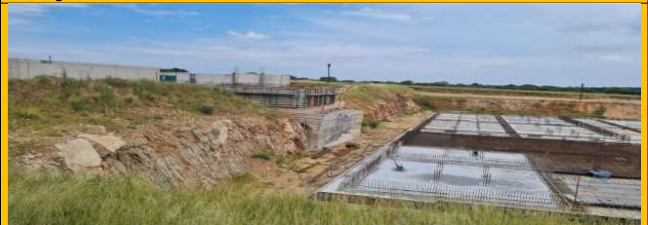
New Regional Wastewater Treatment Plant
