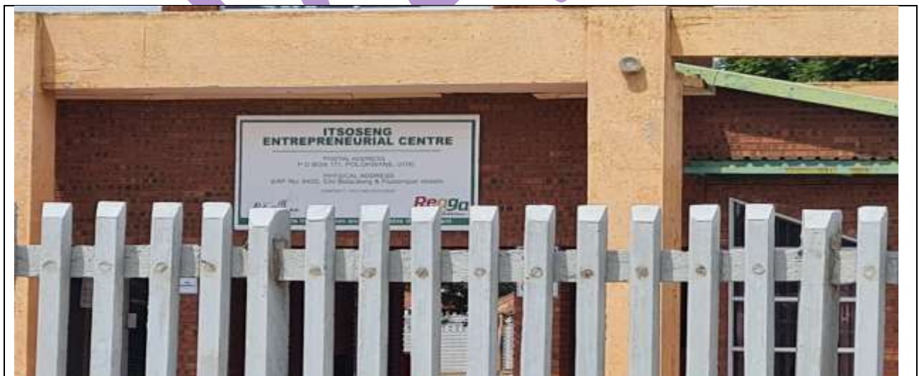
Fencing of Itsoseng Entrepreneurial Centre Completed 1
