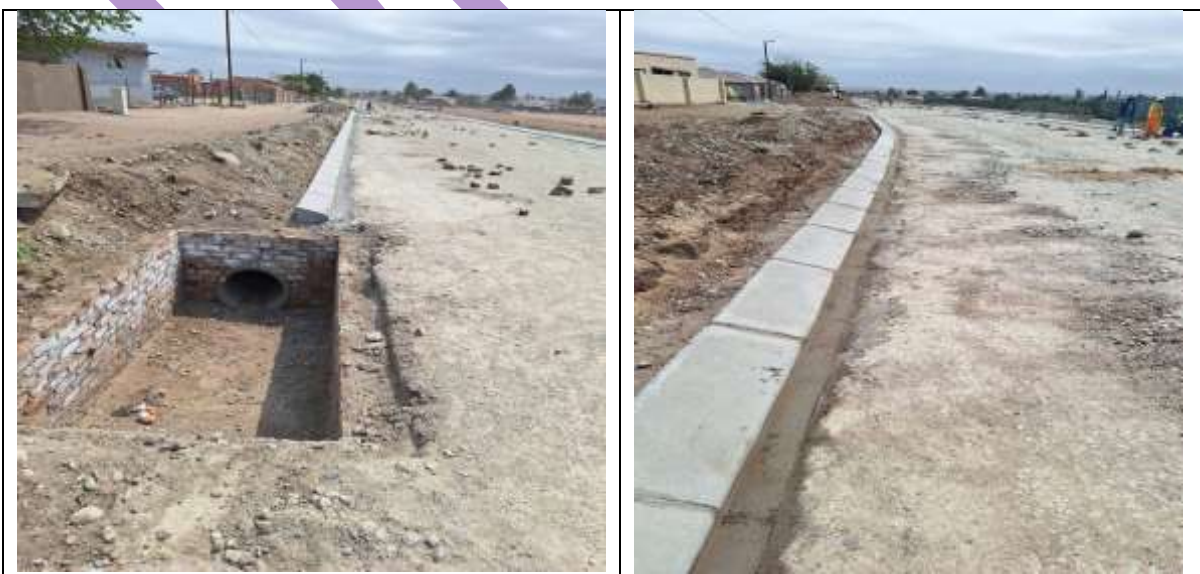
Paving of internal Streets at Seshego Zone 6
