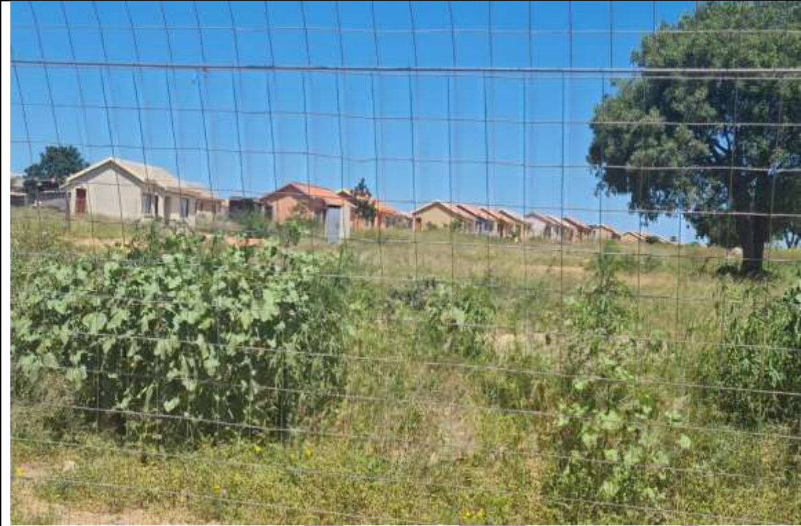
Electrification of Urban Households in Seshego Zone8 Ext. 133 Phase 3.
