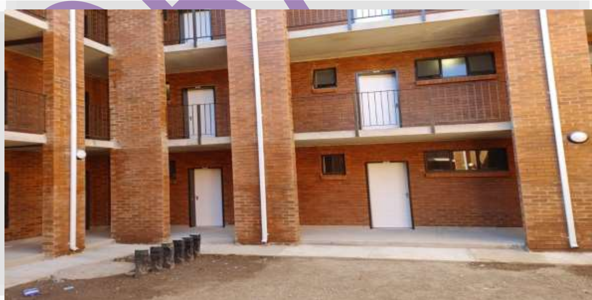
Annadale Ext 2 Completed
