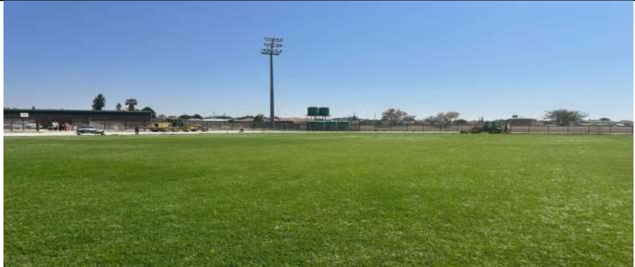
Completed Project -Upgrading of Seshego Stadium
