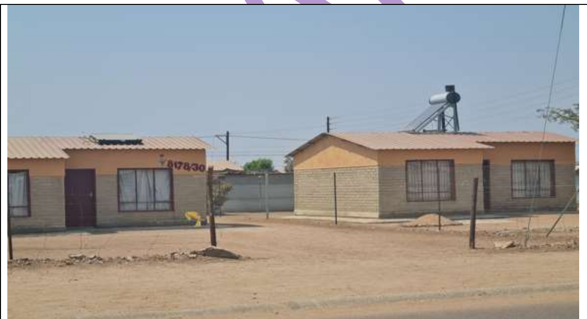
The two types of solar water geysers installed at Mohlakaneng Source: PLK Energy Services Directorate
