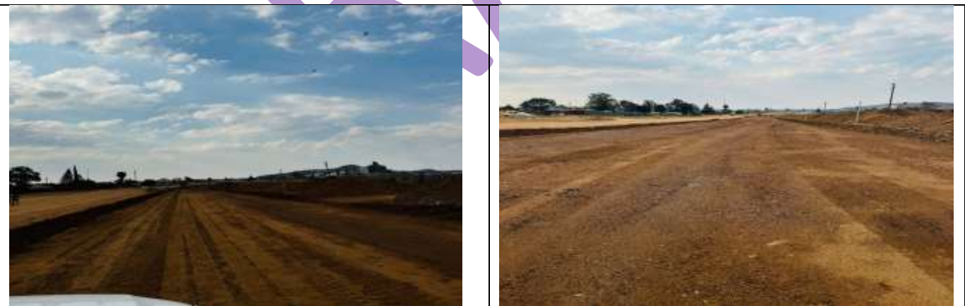
Upgrading of road from Nobody Traffic circle to Moshate
