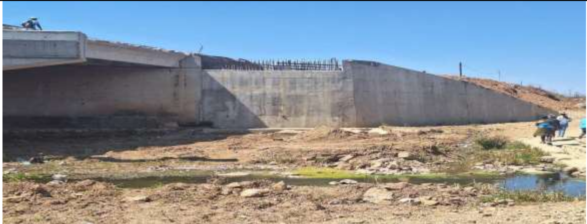
Widening of Sandriver Bridge 2
