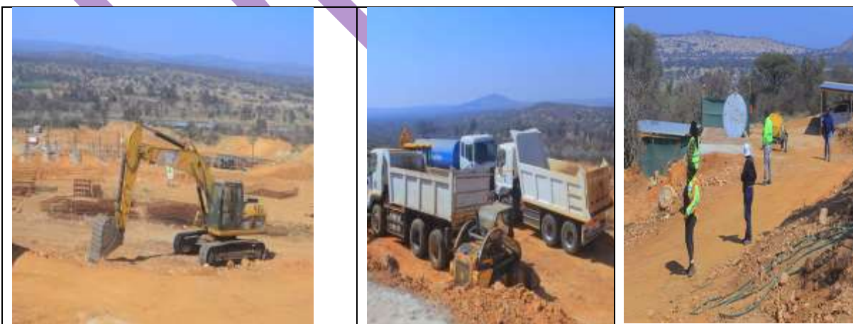
Construction of Limpopo Provincial Theatre (1)
